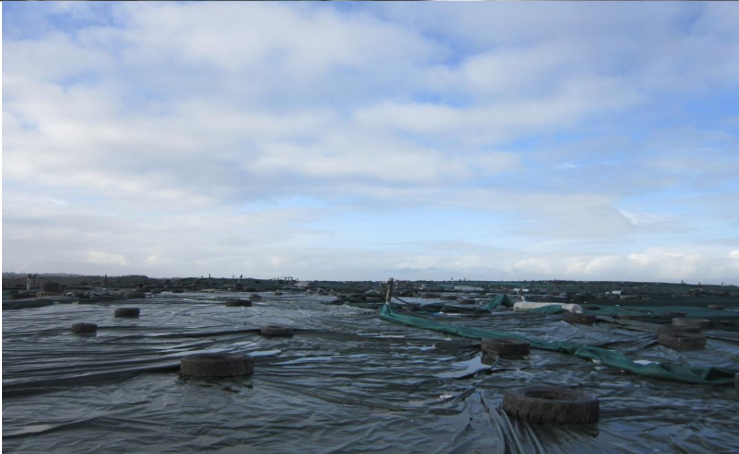
Plate 22: Properly managed waste - Compacted and covered in a modern sanitary landfill, Dublin.
