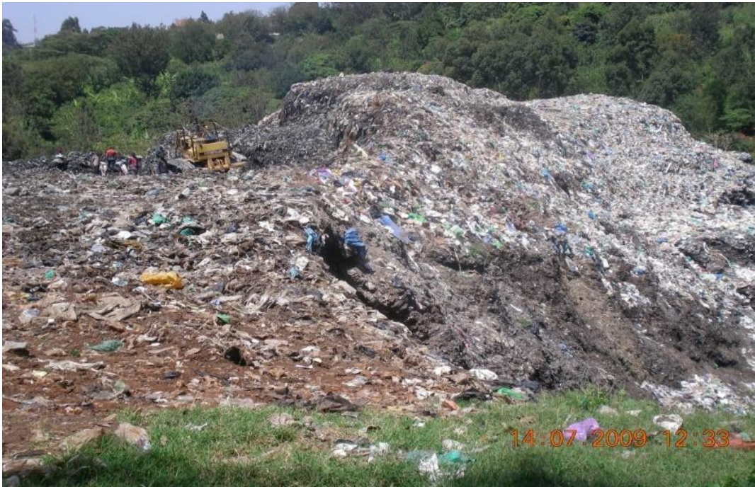
Plate 17: A poorly maintained open dumpsite
