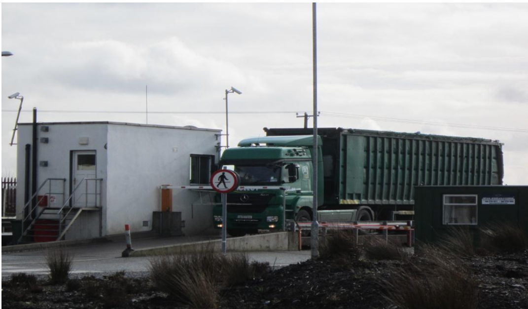
Plate 21: A standardized modern weighbridge at a landfill in Dublin
