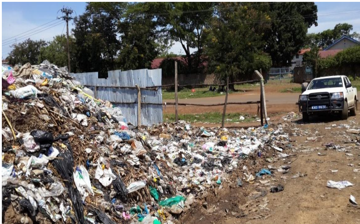
Plate 4: Unmanned wrecked main entrance at the Kachok dumpsite
