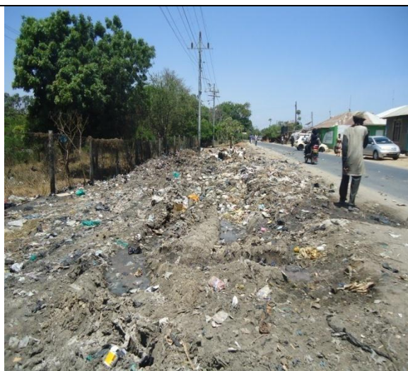
Plate 13: Illegal dumping on a road reserve - a common feature
