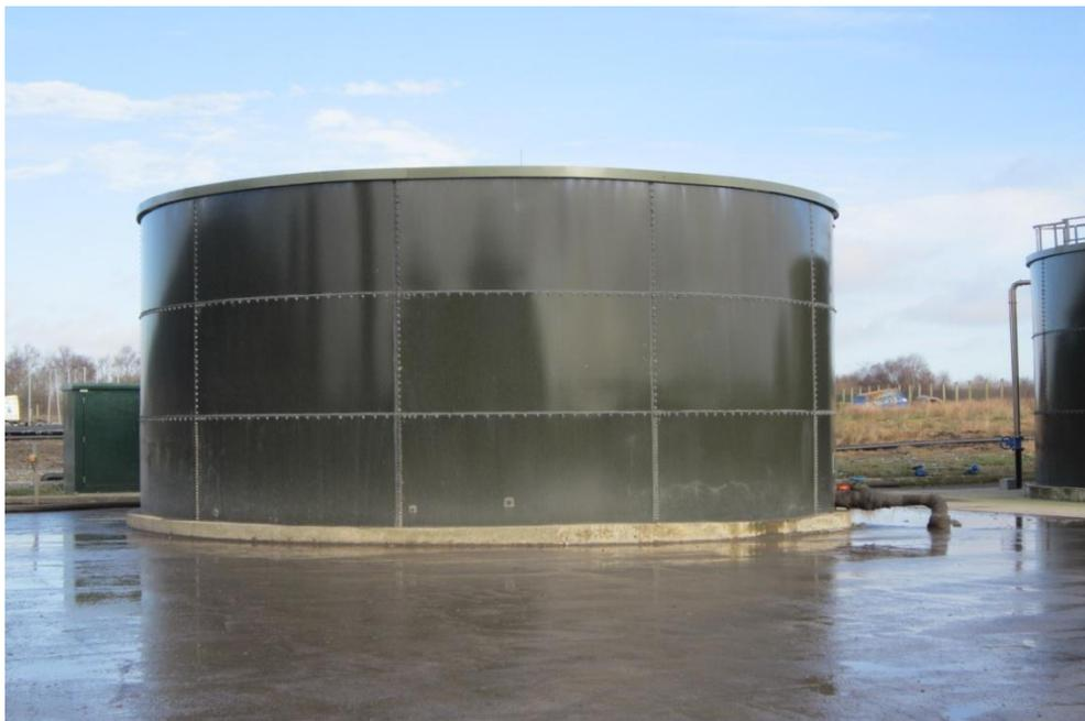
**Plate 23:** A leachate collection system in a modern sanitary landfill, Dublin
