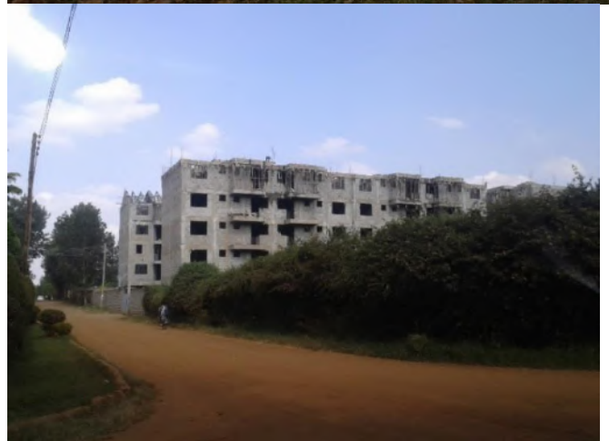
Other similar residential flats under construction near the proposed project site
