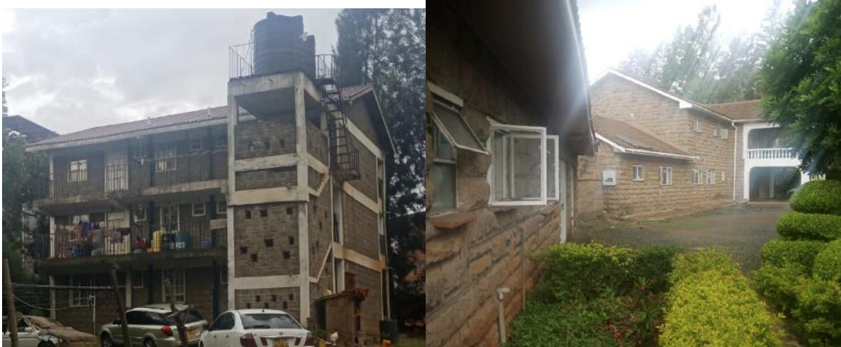
Figure 1: Existing Building Structures at Site
