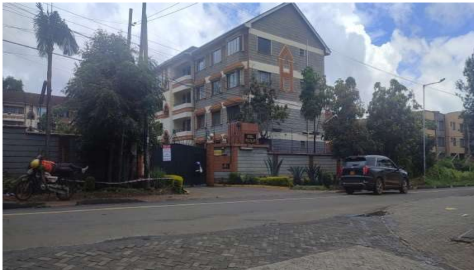
Plate 5: Royal Promenade Apartments neighboring the project site
