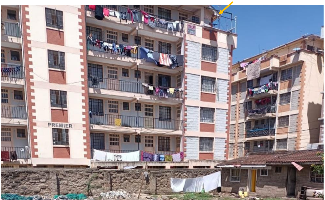
Photo 1: showing similar development behind the proposed site
