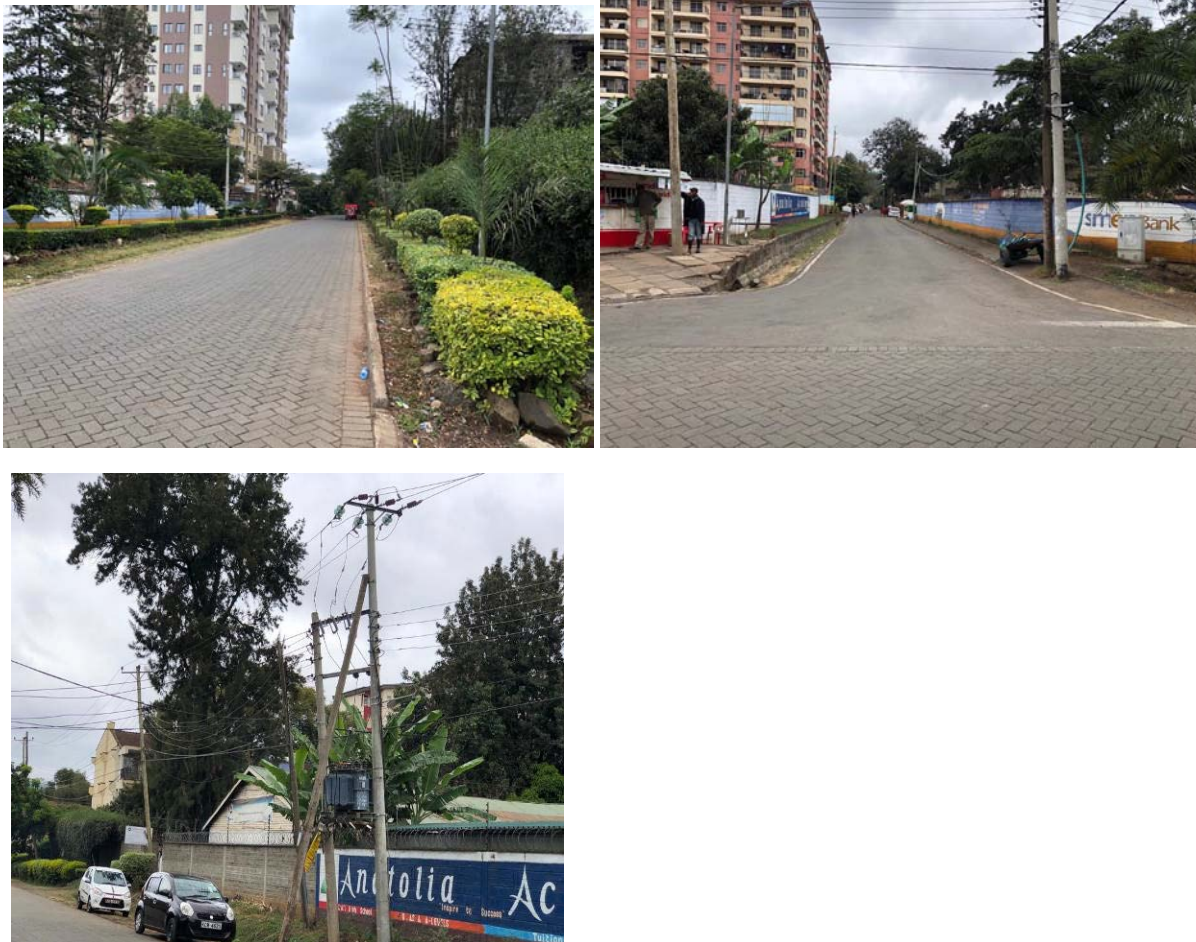
Plate 2: Part of infrastructure in the area
