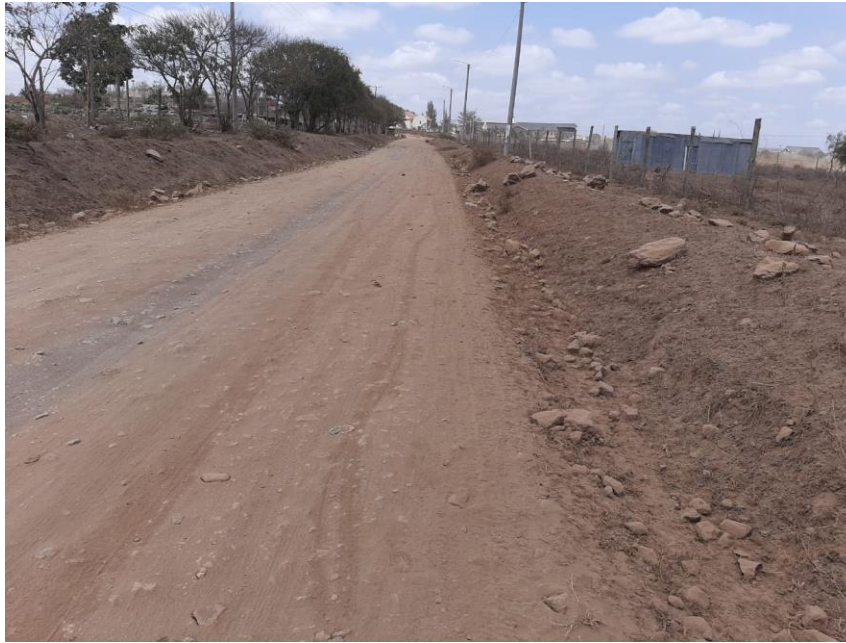
Figure 3: Access road and electricity supply to the project area
