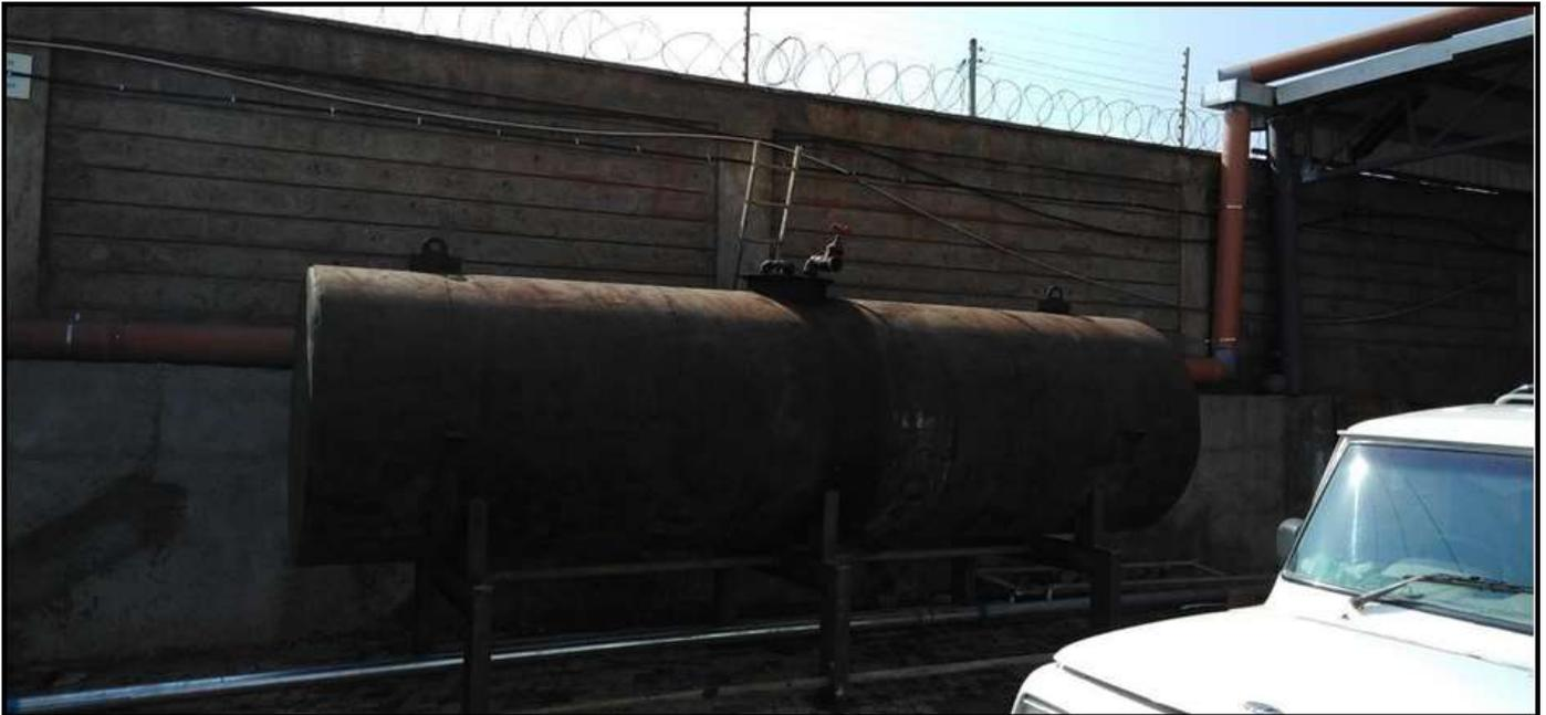
Photo 2: Showing industrial diesel storage tank at the project site for storing bulk diesel for use.
