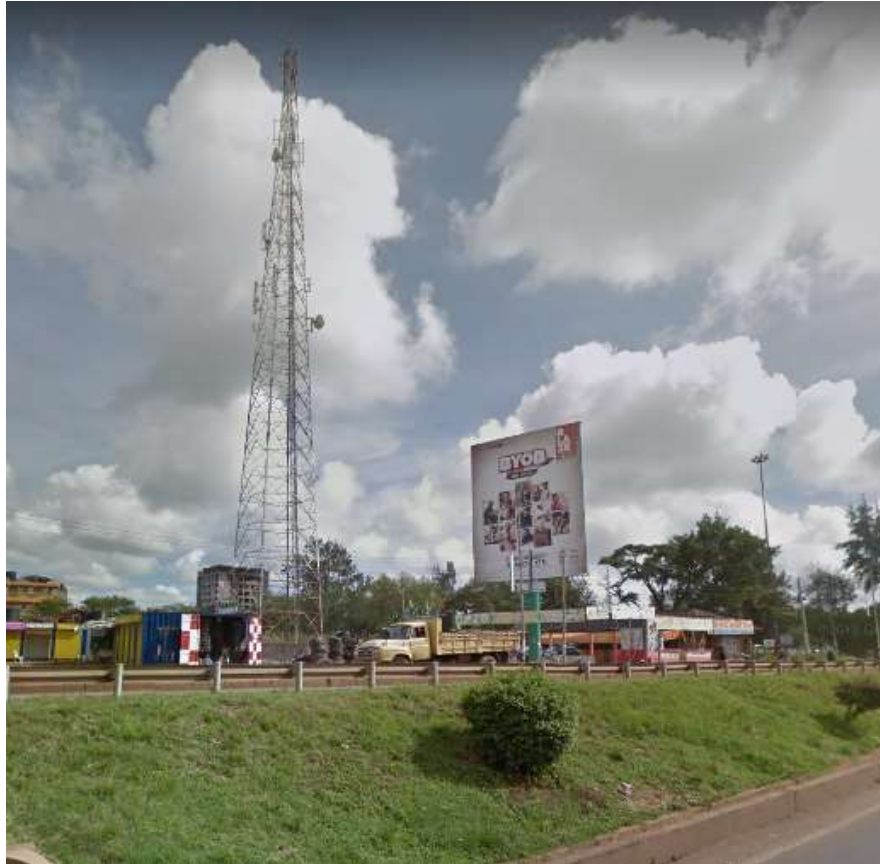
Figure 8: Some of the Telephony Infrastructure in the Area
