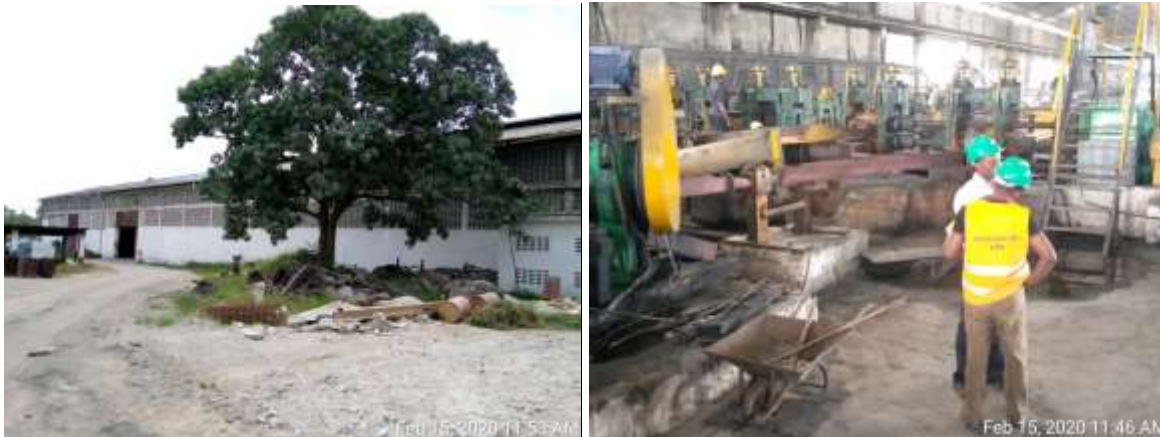
Plate 1: A section of the outside of the godown & the inside shoeing part of the steel mill inside
