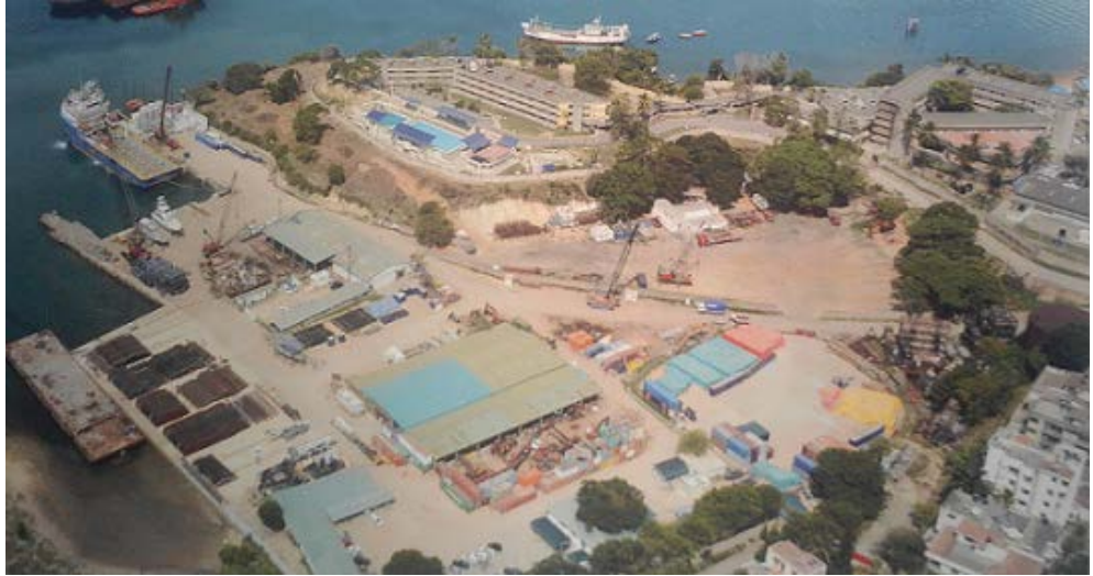
Aerial view of the proposed project site
