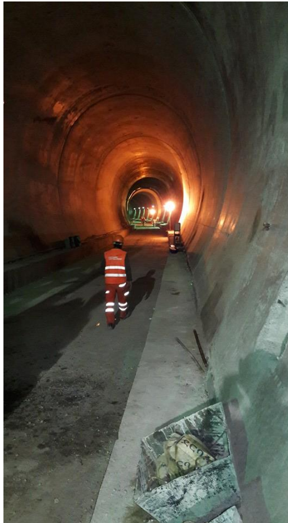
Plate 2- 2: SGR tunnel in the Ethiopia-Djibouti railway project
