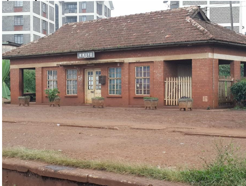
e) Longonot Station
