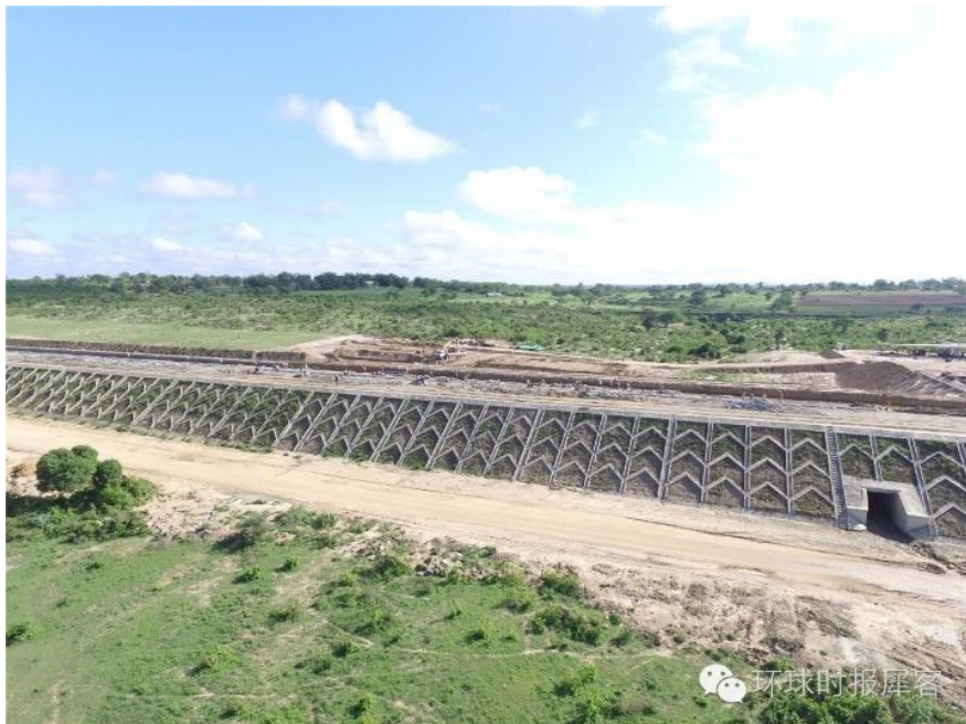
Plate 2- 5: Embankment protection approach used in the SGR-I project
