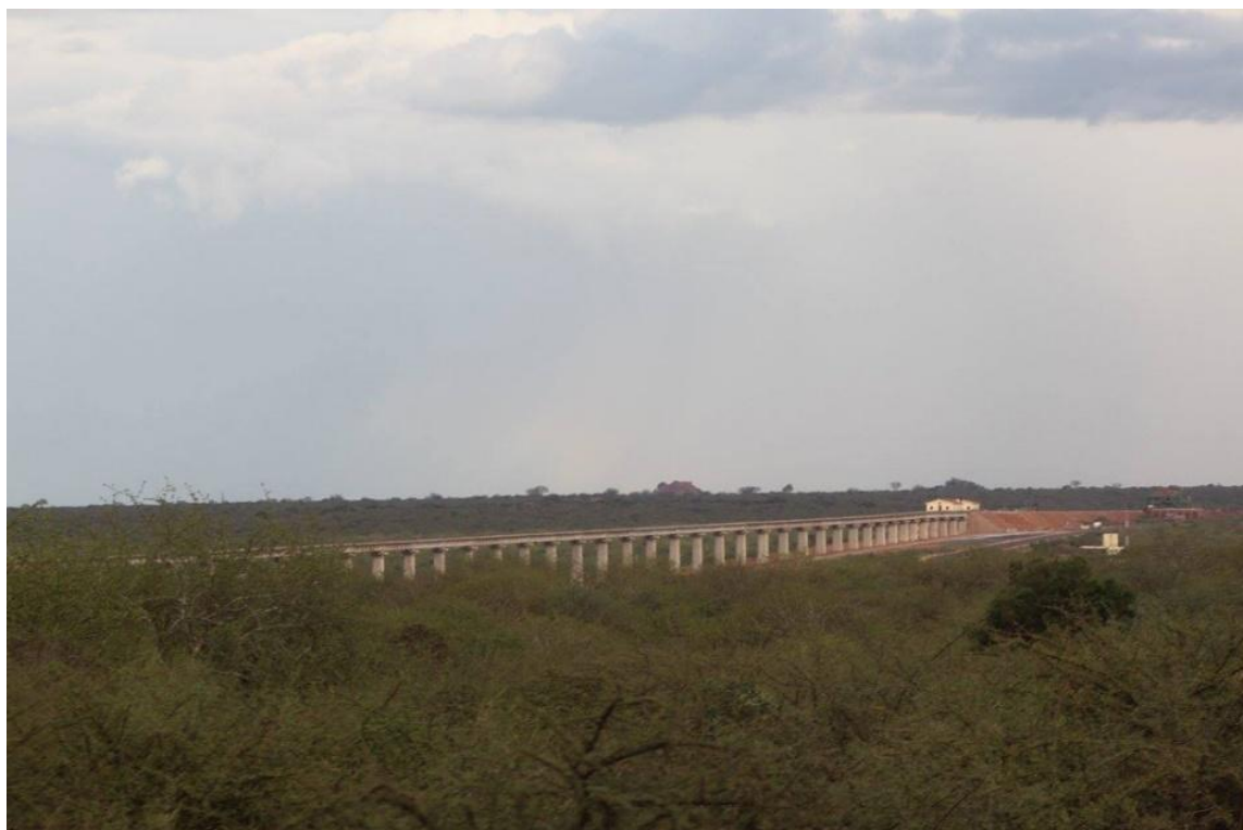
Plate 2- 3: Structure of a SGR underpass bridge in the Phase I project
