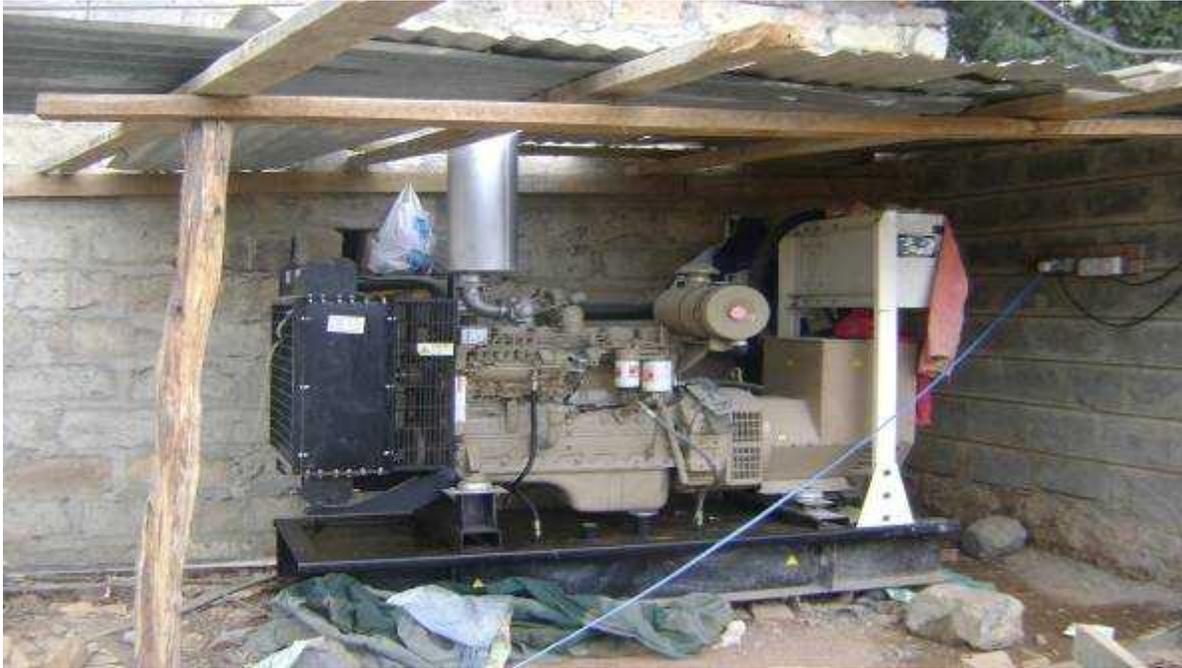
Fig 3 Standby Generator at proposed site
