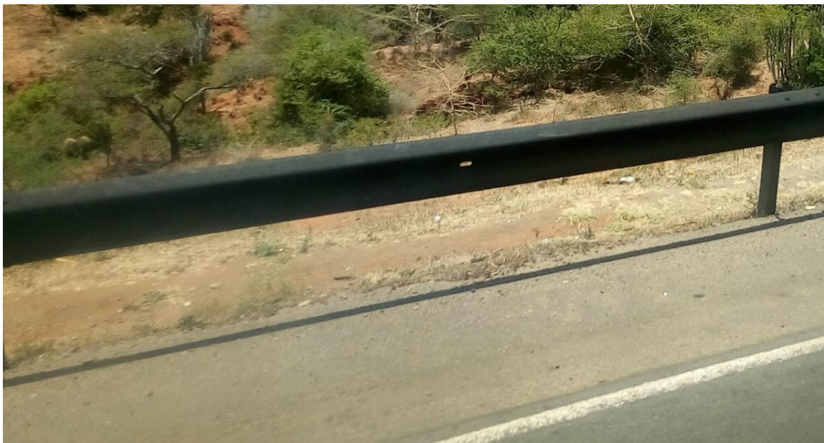
Figure 58: Black emissions on Guard Rails.
