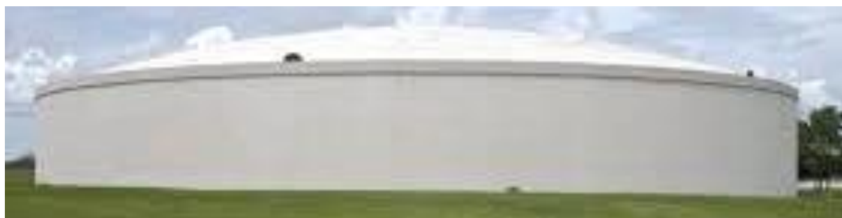
Figure 6: Example of 5 million litres gallons tank.
