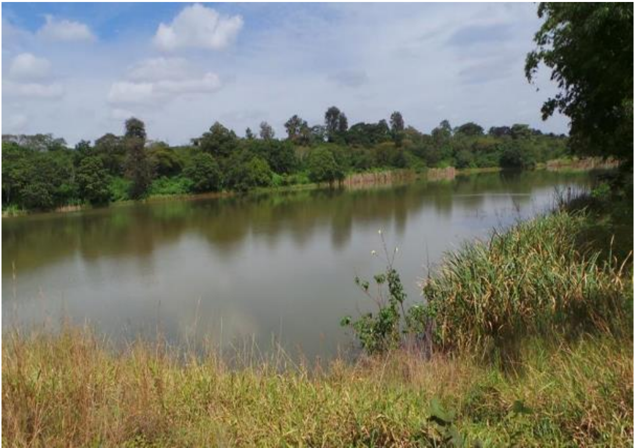
Plate 3-2 A section of the Comte earth dam at the proposed Tatu City Extension (Mchana Estate)
