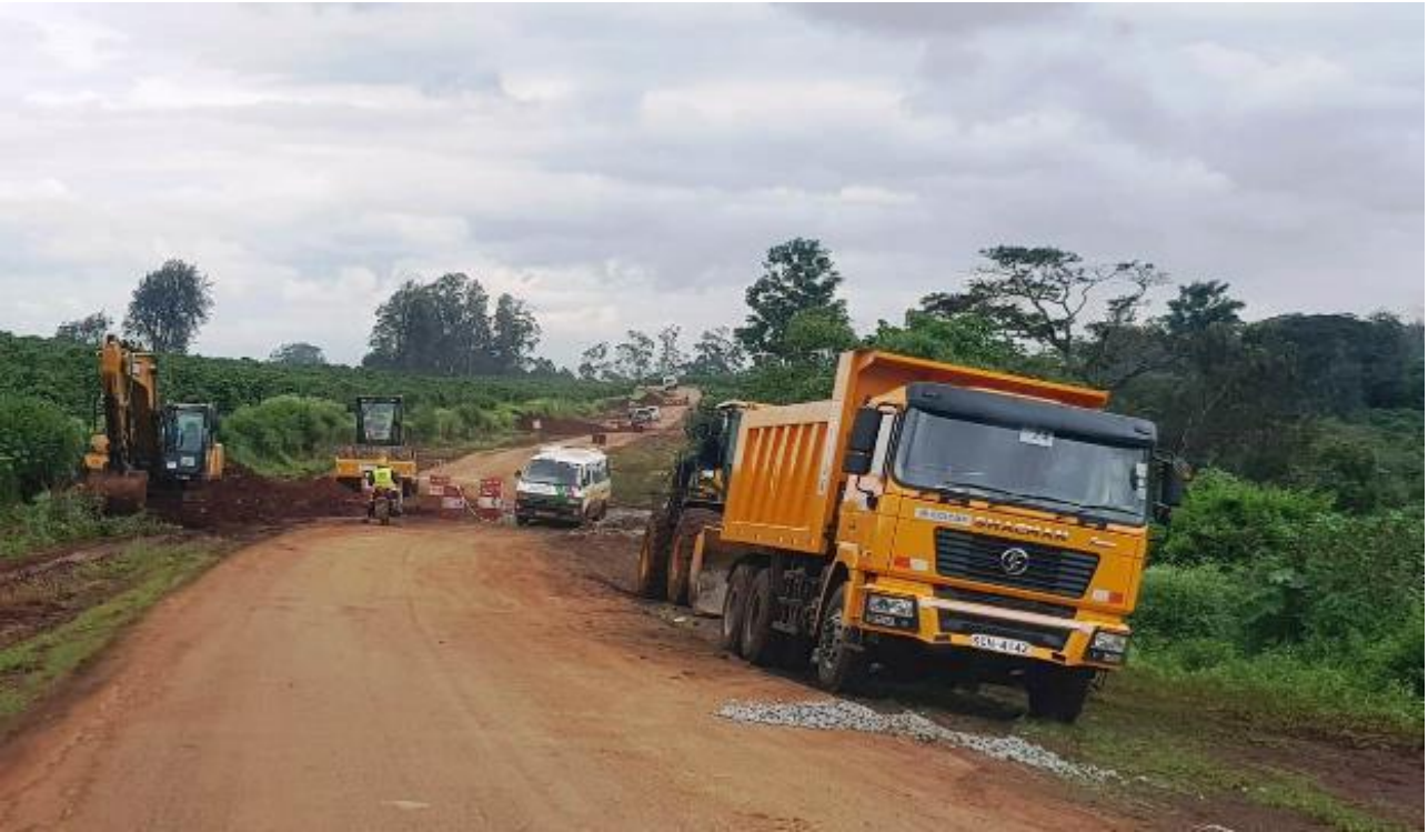
Plate 3-23 Road construction works along Ruiru – Githunguri Road (C65)
