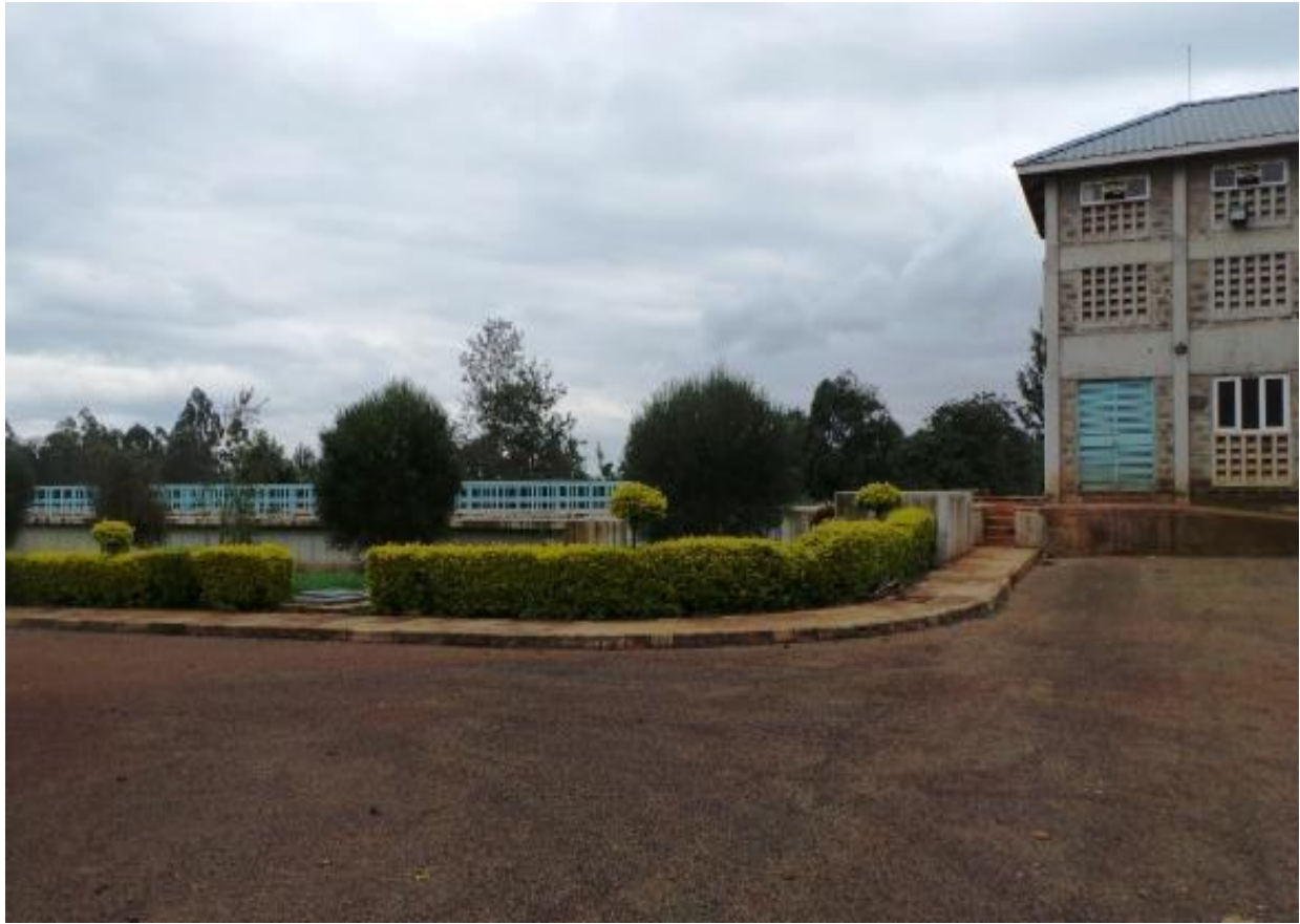
Plate 3-5 RUJUWASCO Offices and plant located at Tatu City Phase 1
