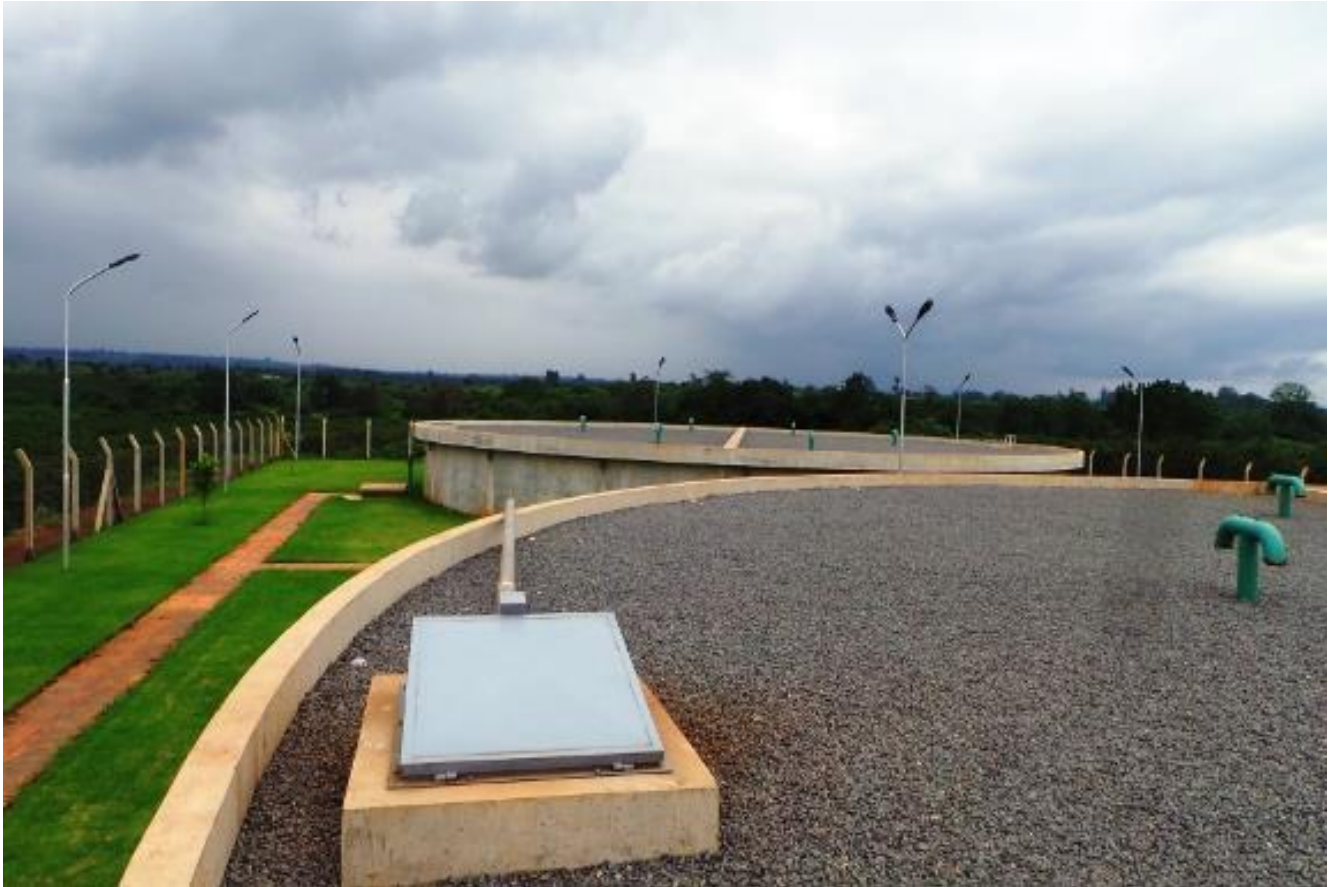
Plate 3-6 Water treatment and Storage plant
