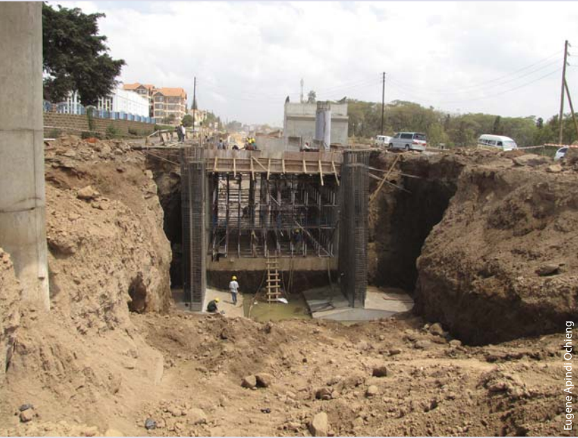
Construction of an underpass at Pangani.
