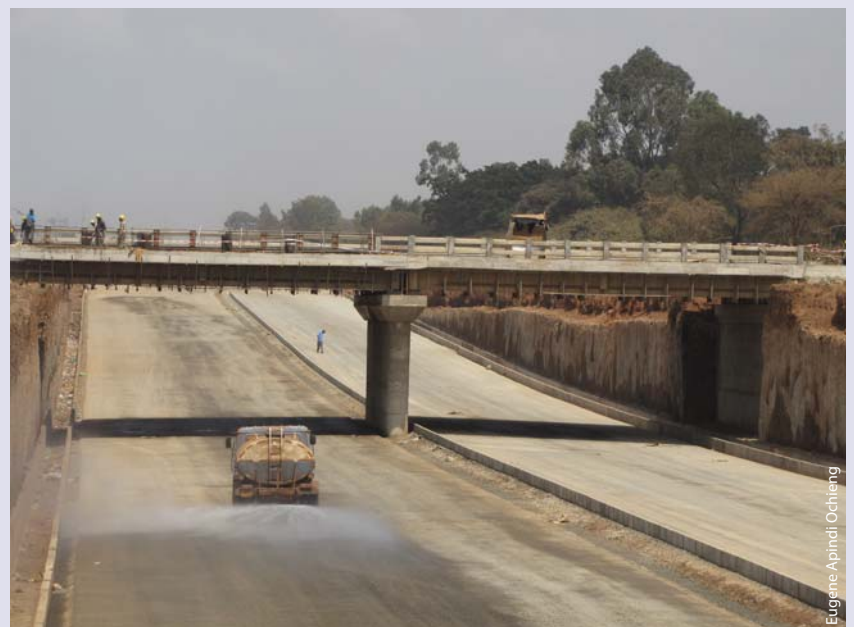
An overpass by GSU headquarters connecting the Thika and Outer Ring roads.
