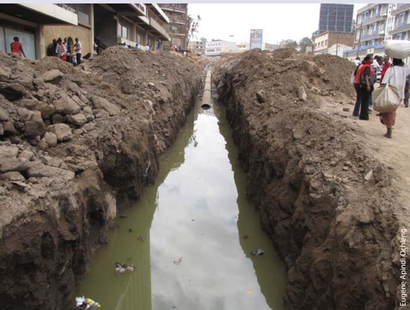
A major sewerline under construction at Ngara.
