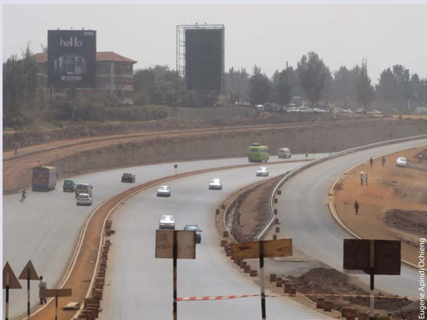
A panoramic view of a completed section of the Thika Superhighway.
