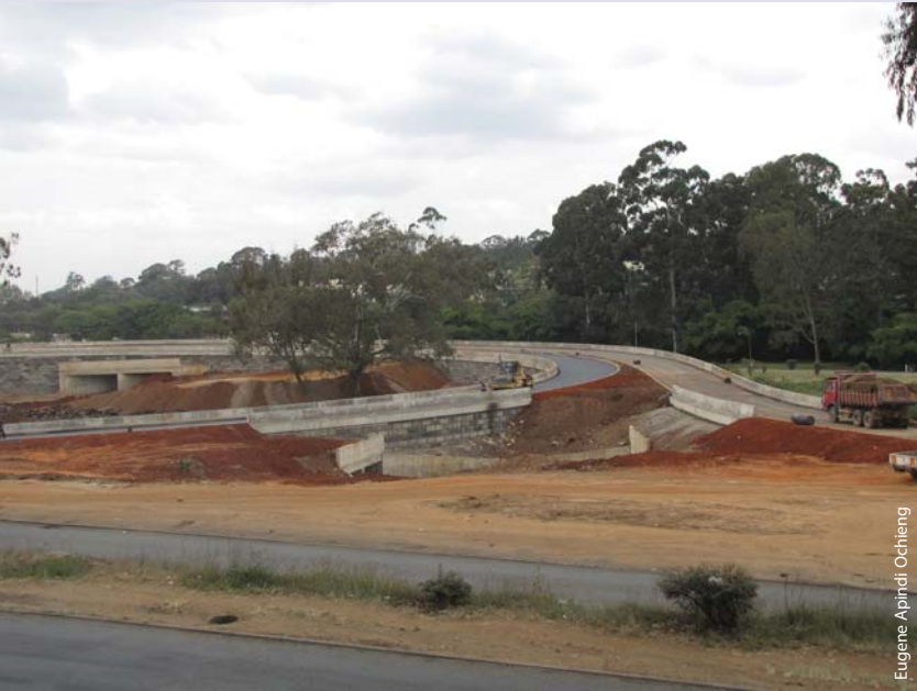
The Museum Hill/Uhuru Highway interchange.
