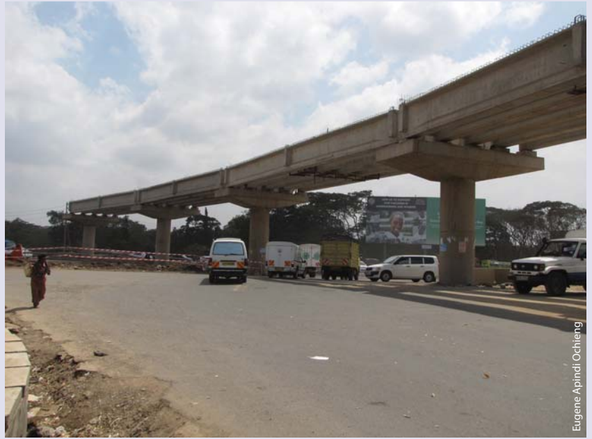
Construction of a flyover at Pangani.
