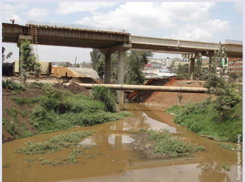
A flyover above the Nairobi River at the Globe Cinema roundabout.
