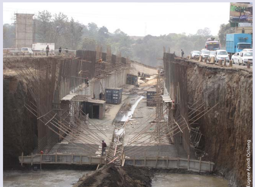
Construction of an underpass at Pangani.
