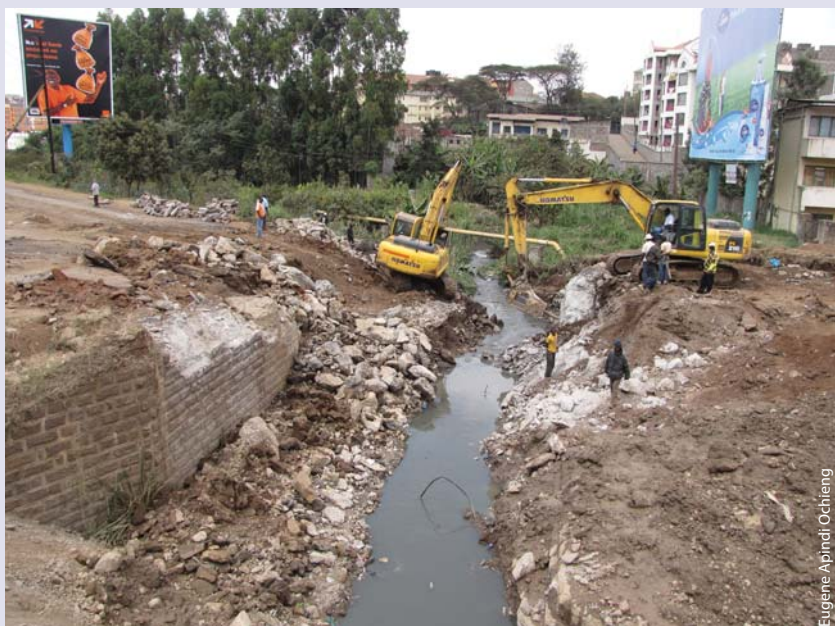
Excavation works for bridge construction over the Pangani/ Muthaiga River.
