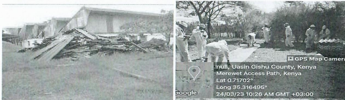
Poorly managed asbestos: A licensed transporter preparing to transport the removed asbestos waste for disposal
