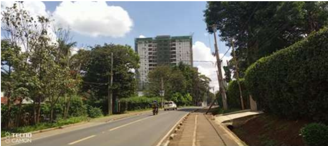
Photo 3: Showing site accessibility off Riverside Drive, Westlands area.
