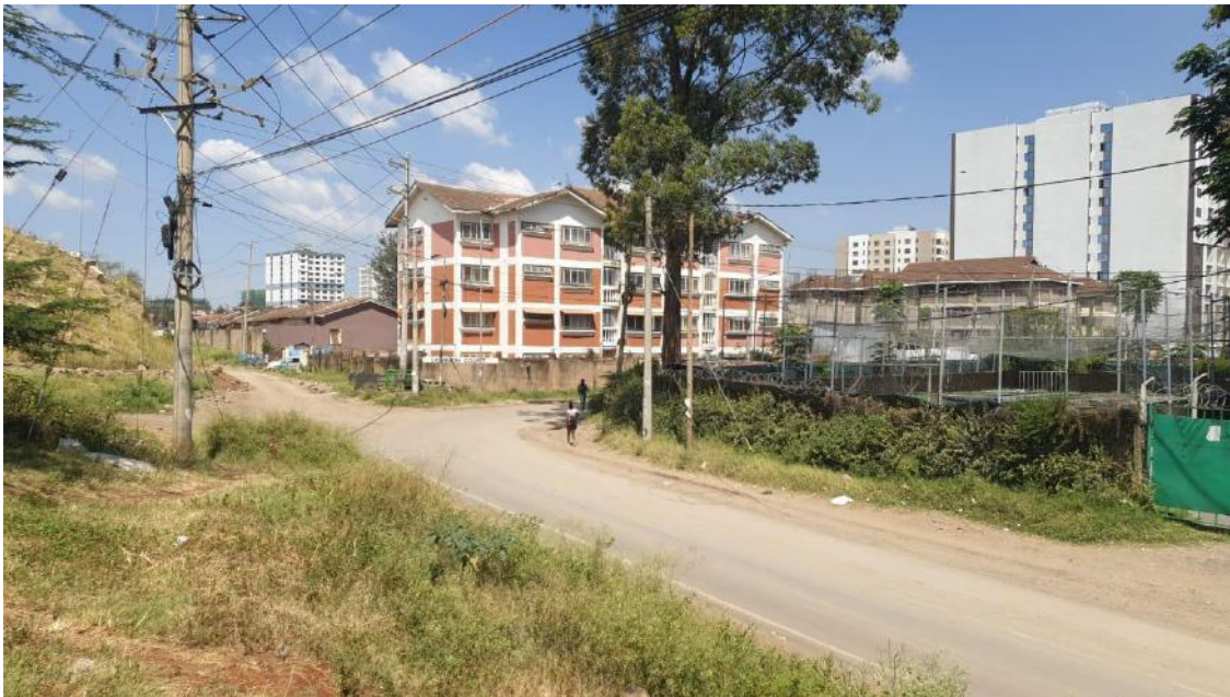
Plate 4: Dominion Court, a 4-storey residential flat direct opposite the site
