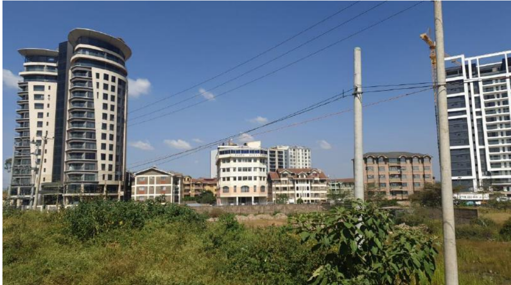
Plate 5: Five storey Allimex Plaza adjacent to The Curve
