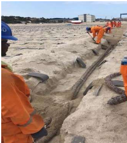
FIGURE 15 - INSTALLATION OF PVD AT PORT
