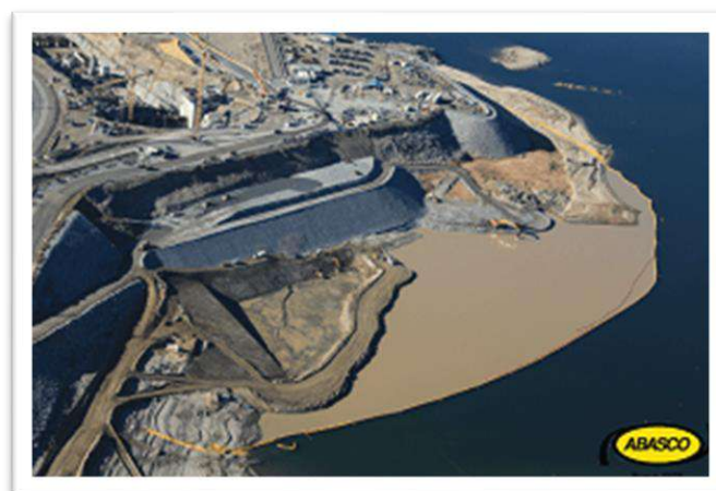
FIGURE 142 – TURBIDITY CURTAIN USE IN MARINE CONSTRUCTION
