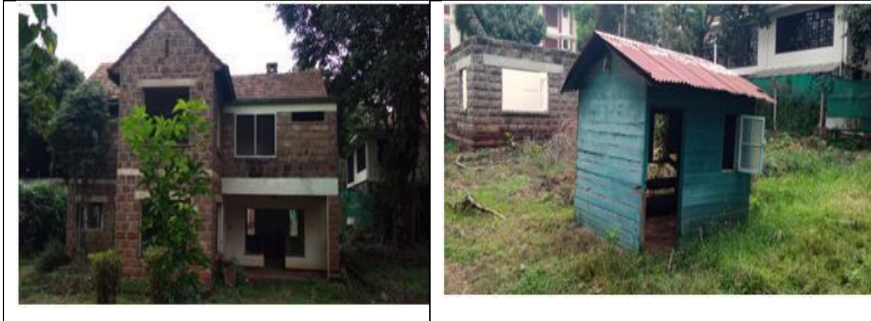
Figure 4: Current status of the project site
