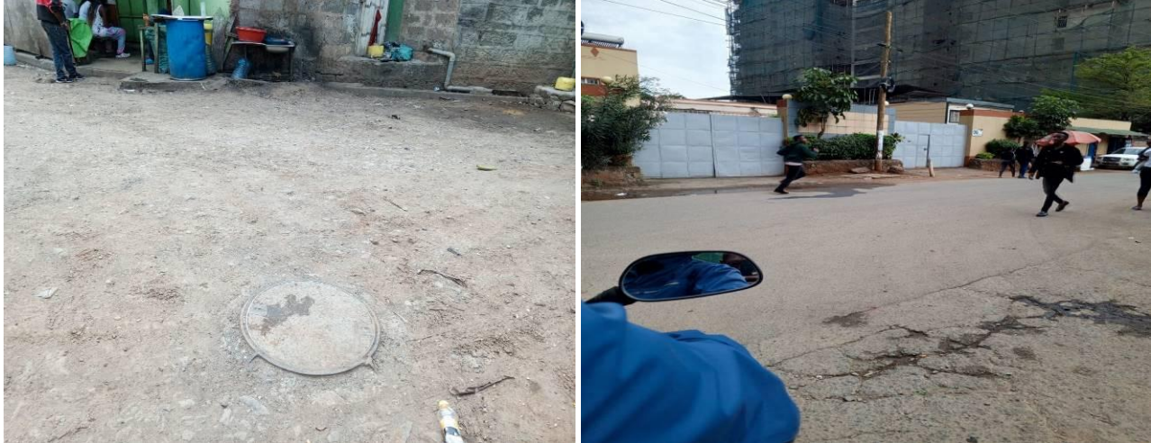
Plate 1: Part of infrastructural development in the area
