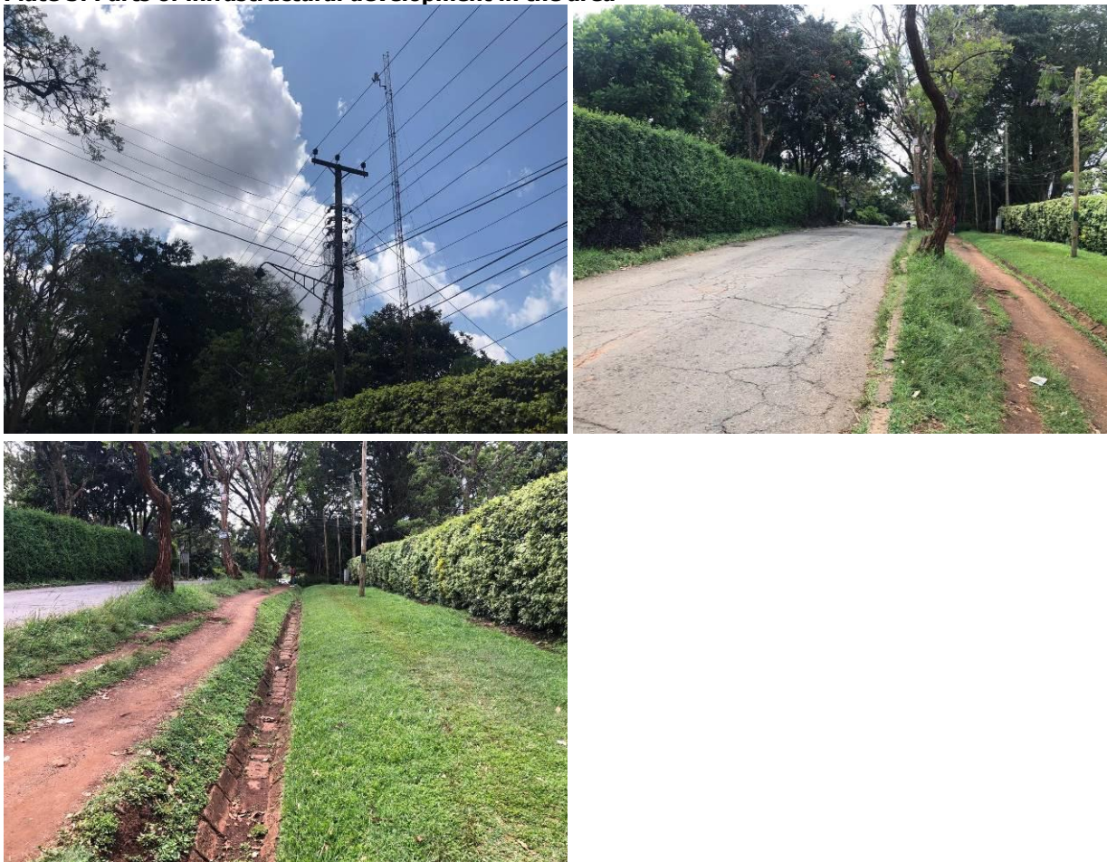
Plate 3: Parts of infrastructural development in the area
