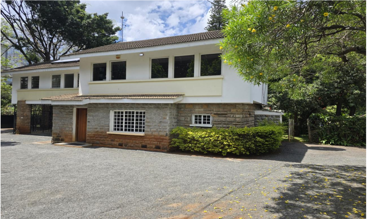
Plate 2: Proposed construction site with a house to be demolished (source; field survey)
