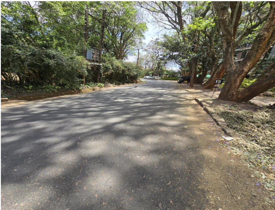
Plate 3: Access road from Brookside Groove. Matundu Lane (source; field survey)
