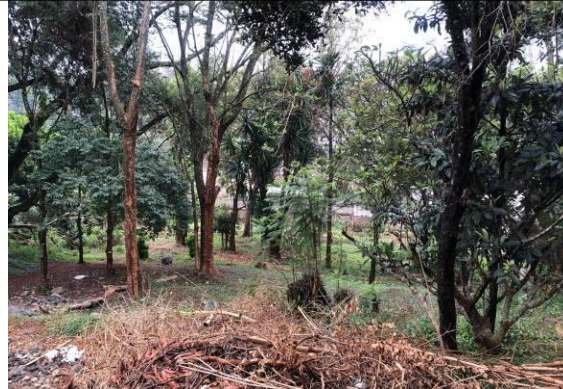
Part of the proposed site with structures to be demolished to pave way to the proposed project
