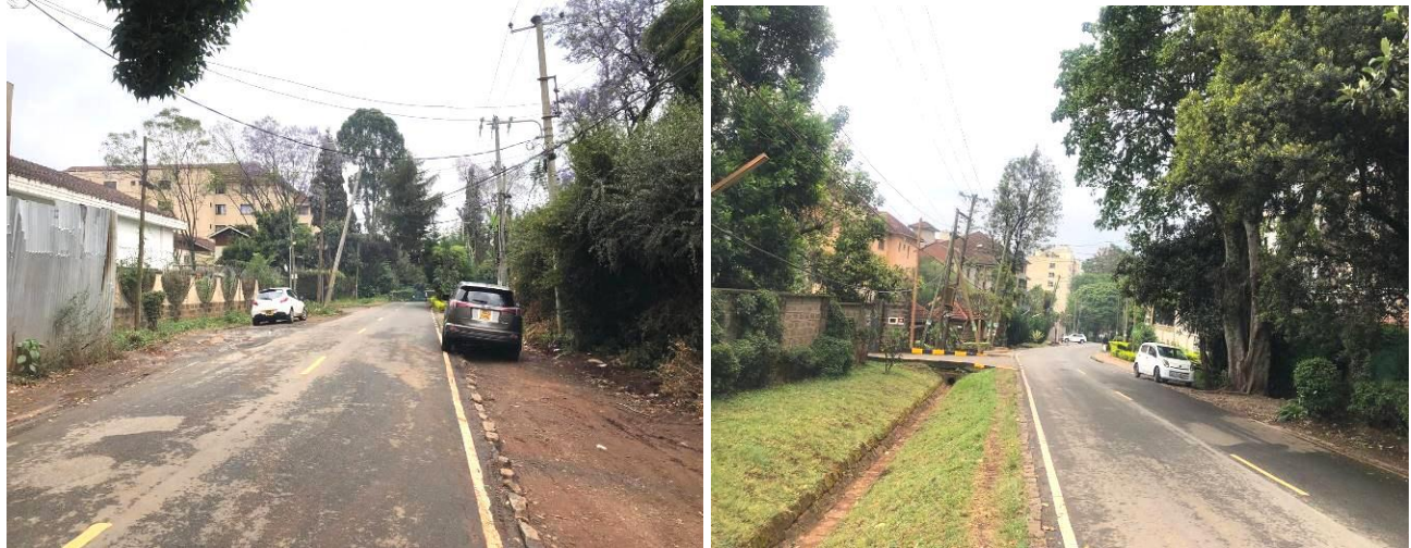
Plate 3: Parts of infrastructural development in the area
