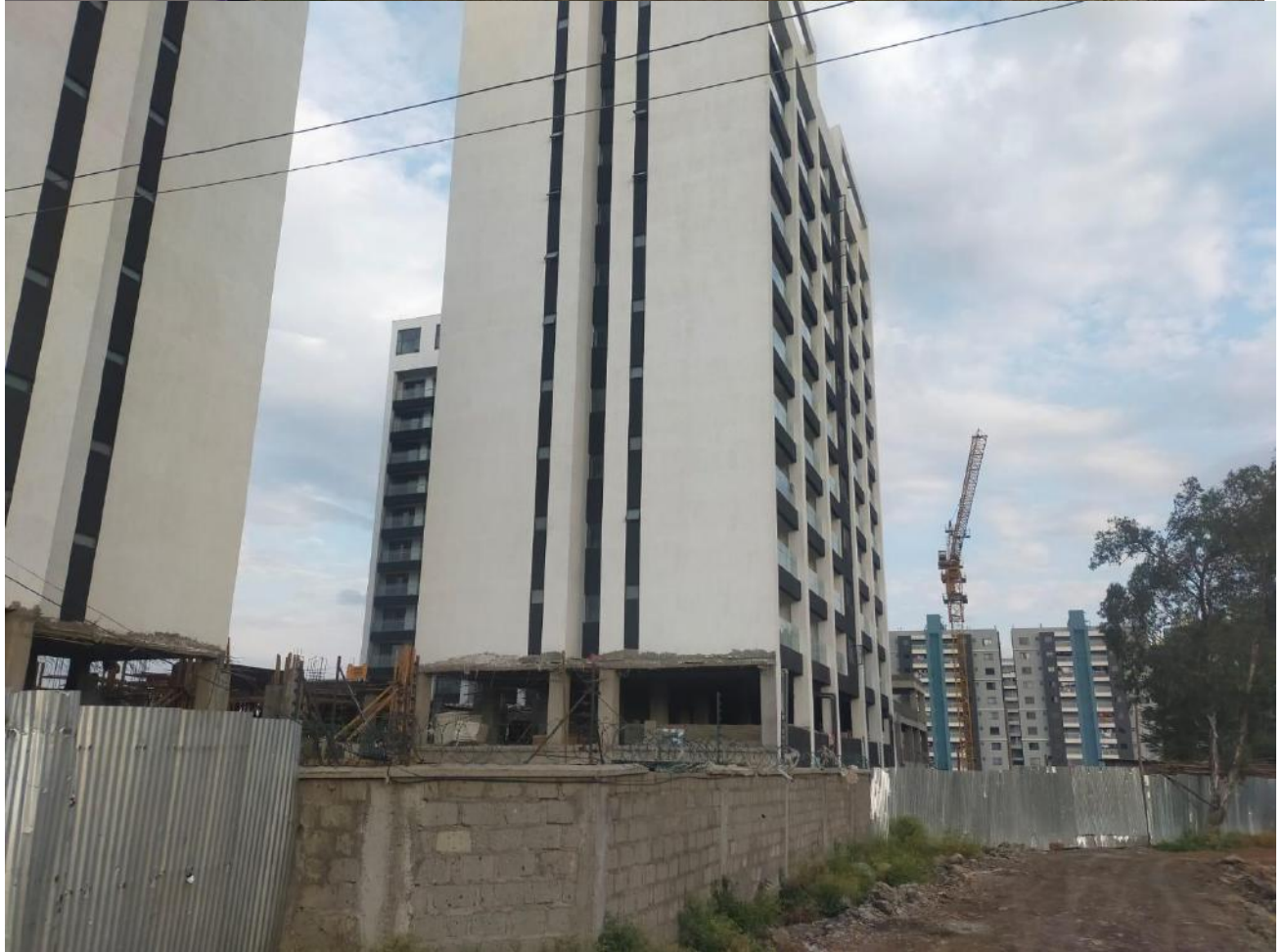
Ongoing construction of residential apartments in the vicinity
