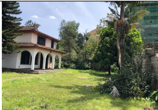
Part of the proposed site with structures to be demolished to pave way to the proposed project
