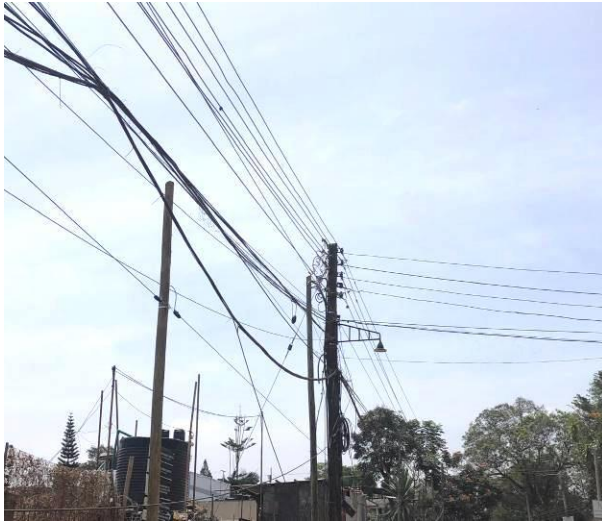
Source: Site Survey
