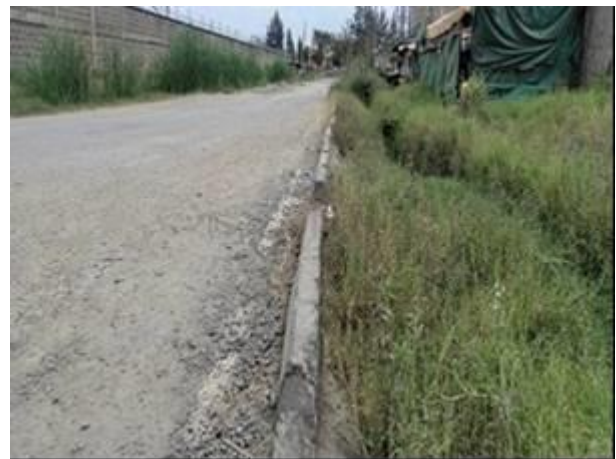
Plate 52: Provision of Roadside Kerbs along the Project Road
