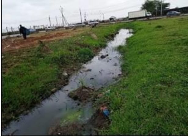
Plate 12: Open Drain along the Median at the Taj Mall U-Turn section
