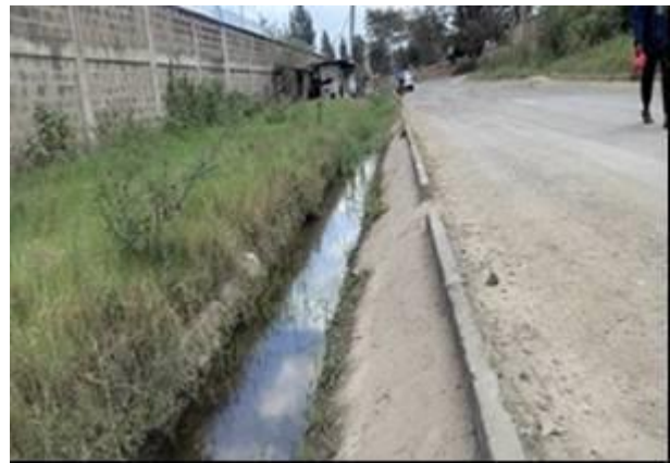
Plate 50: Drainage along the Project Road
