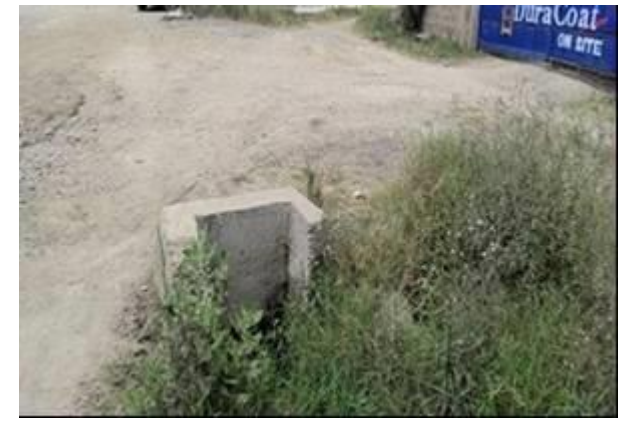
Plate 51: Provision of an Access Culvert along the Project Road
