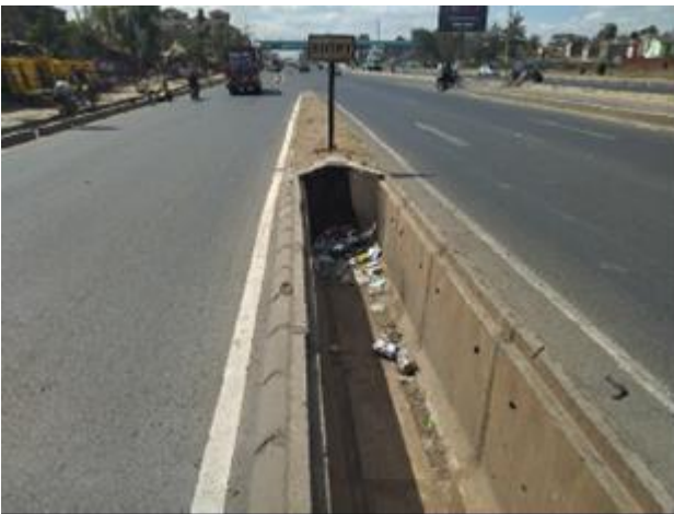
Plate 14: Lined Drains Installed along the Median
