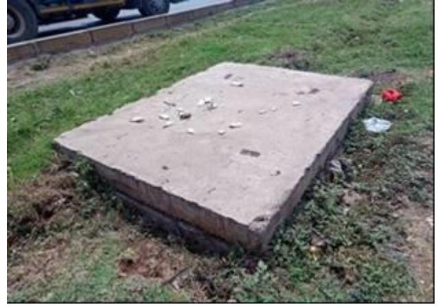
Plate 13: Underground Drainage manhole along the Median
