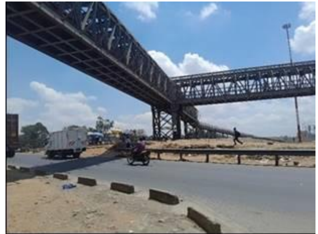
Plate 9: Pedestrian Footbridge at the proposed Allsops Station
