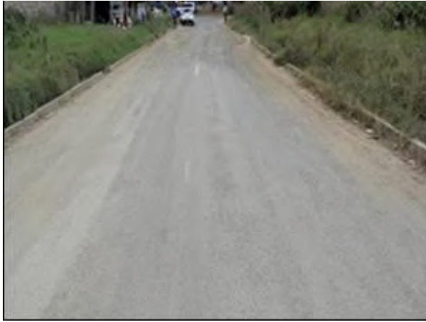
Plate 48: The Project Road has a Bitumen Surface
