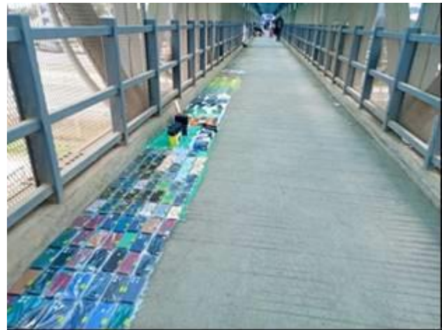
Plate 11: Encroachment on Pedestrian Footbridge hindering proper use
