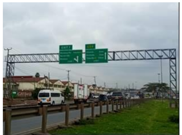
Plate 17: Support System for Road Name Signage Installed along the Median
