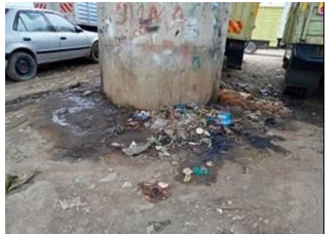
Plate 35: Open Dumping and Defecation along the Median
