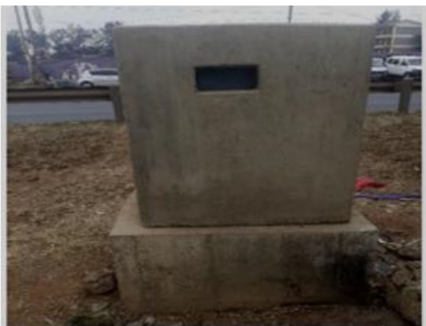
Plate 16: Electrical Circuit Box Installed along the Median
