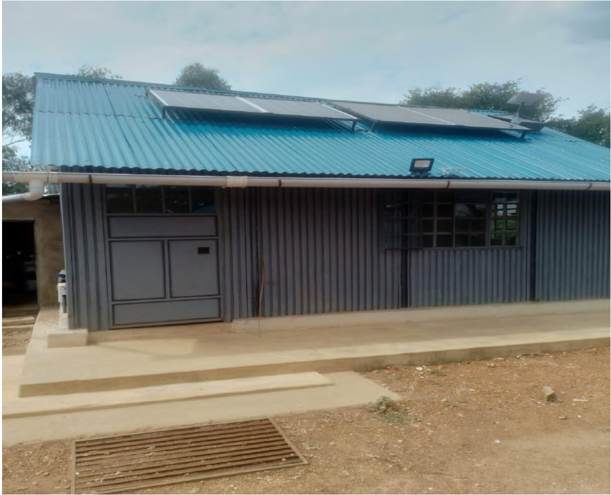
Plate 3.1: Temporary office with solar panel installed at the project site
