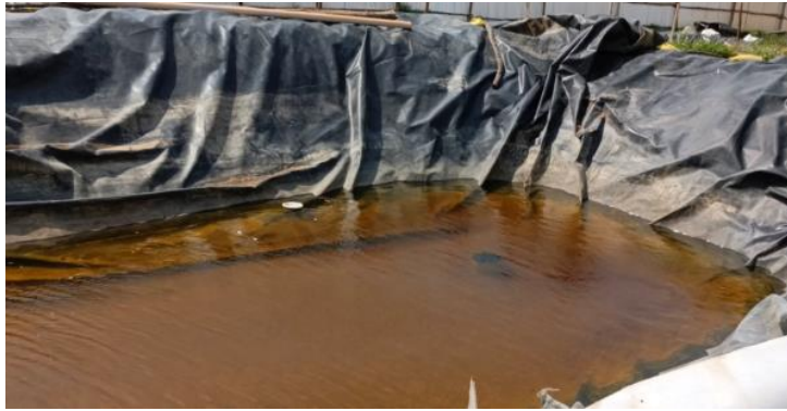
Image 4.3: Leachate collection pond
