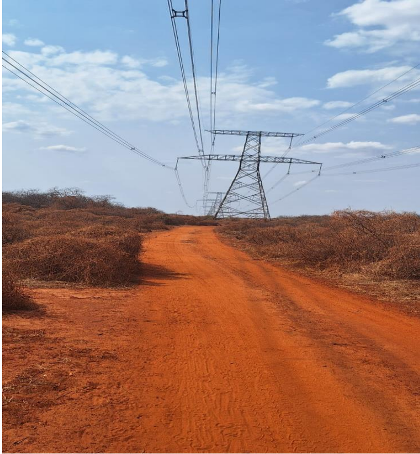
Access and power supply
