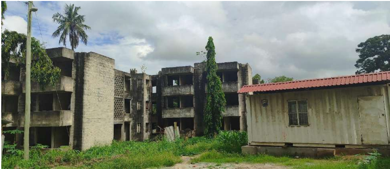
Plate 4-3: A view of the vacant blocks
