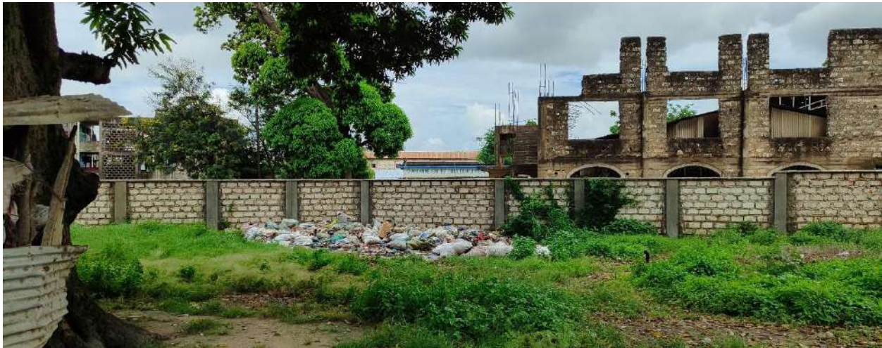
Plate 4-11: A view of the waste holding area
