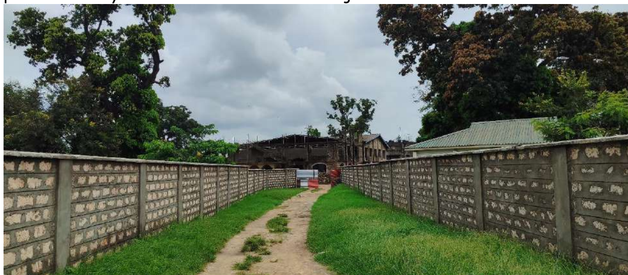
Plate 4-5: A view of part of the perimeter wall.
