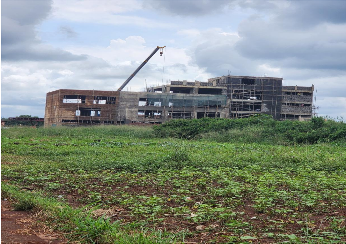
Plate 4:neighbourhood developments - ongoing construction (Astrol Petrol Station)
