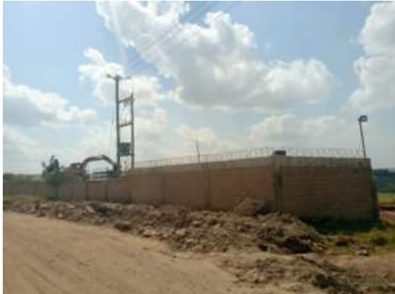
Stone crushing site
