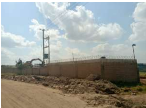
Stone crushing site
