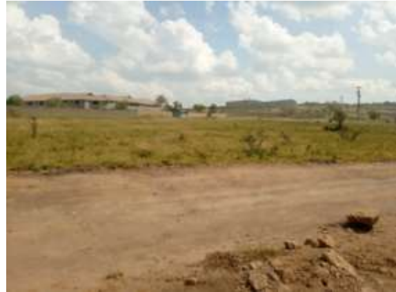
Non-operational school structure
