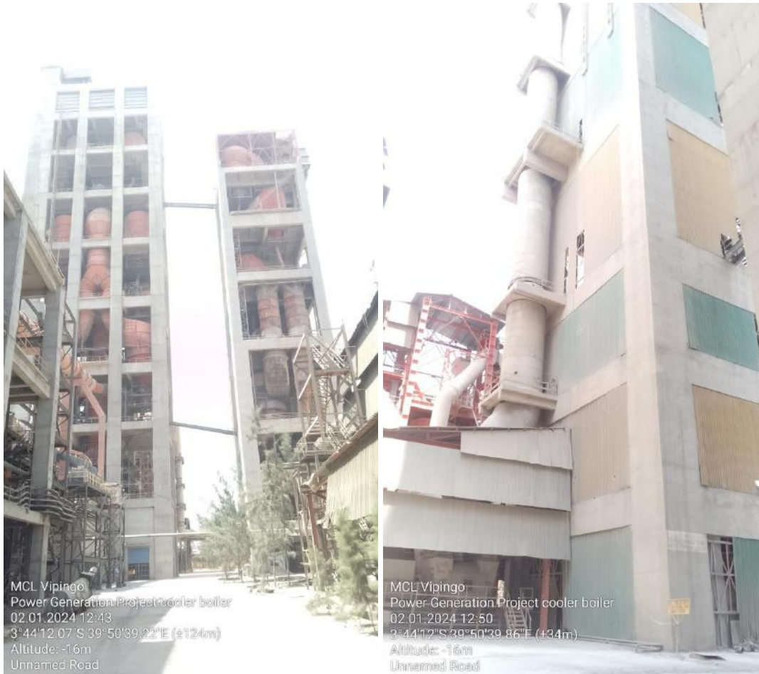
Plate 1 Section were waste heat will be tapped from within MCL Vipingo plant
