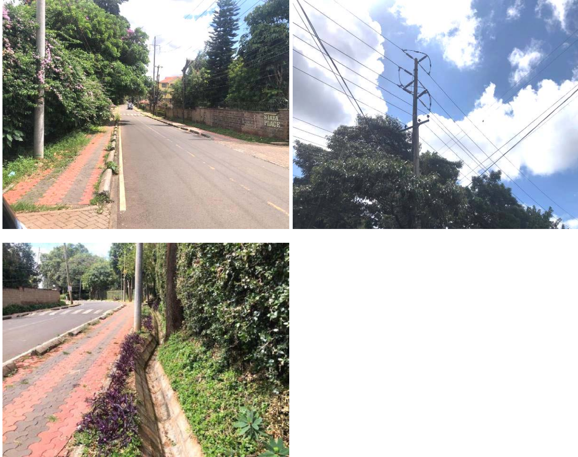
Source: Site Survey
