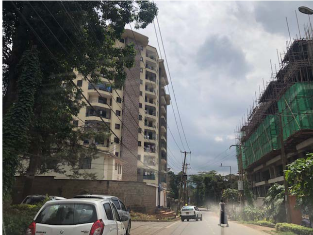
Source: Site Survey
