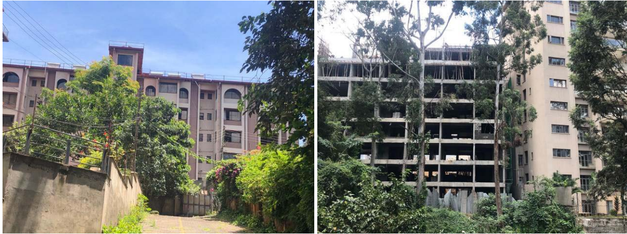
Source: Site Survey
