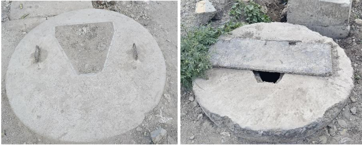
Plate 4: Existing MAVWASCO sewer line manholes in the area
