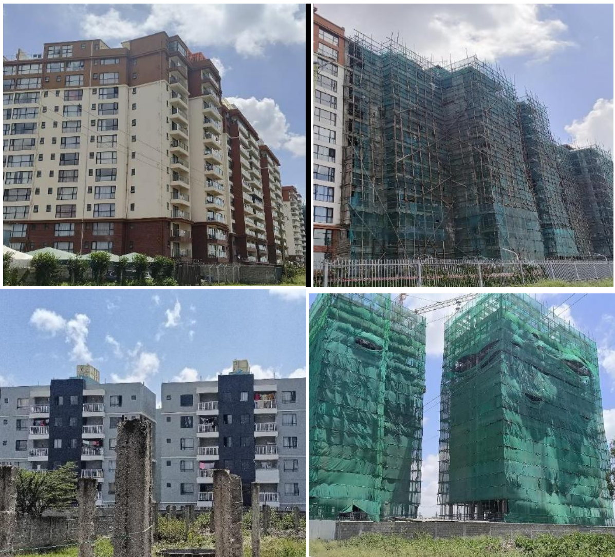
Plate 1: Completed and ongoing residential projects within the project area.
