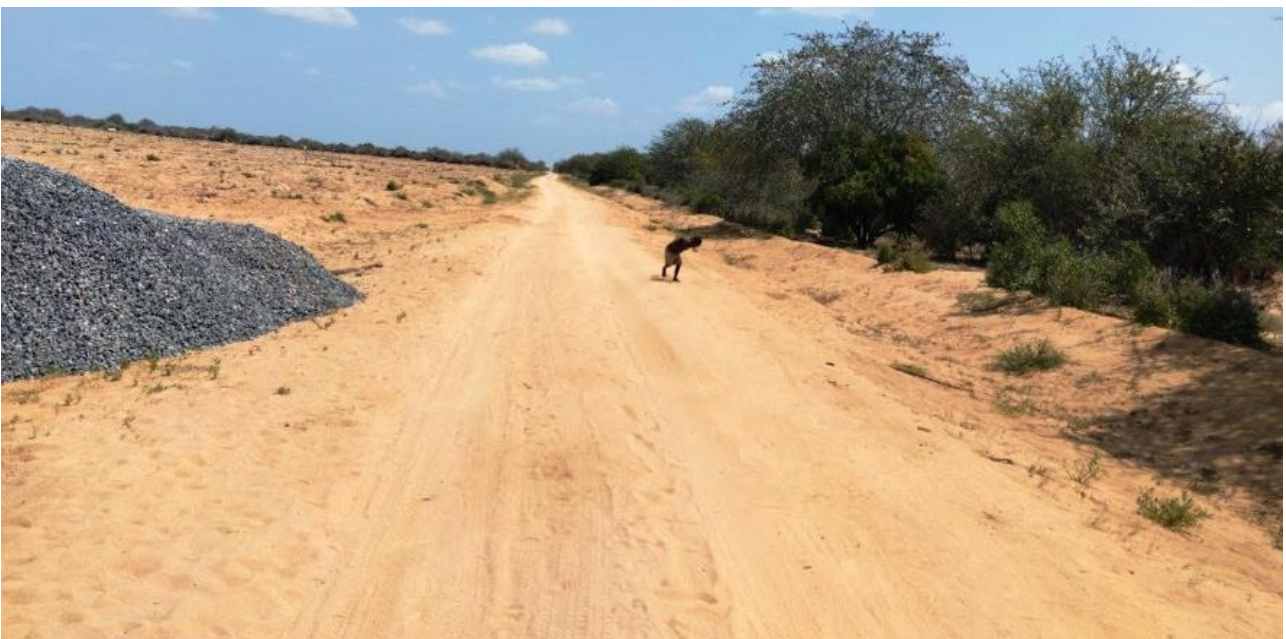
Figure 3: Site access road.
