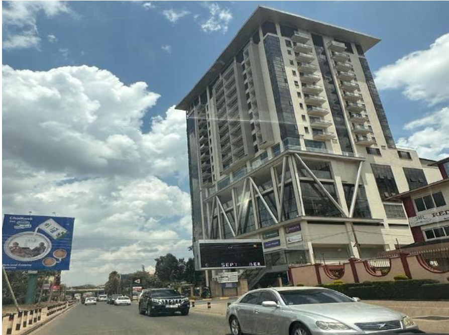
Photo 3. Infrastructure in the area
