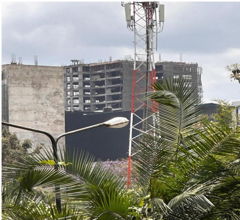
Photo 4. Similar project under construction within the area
