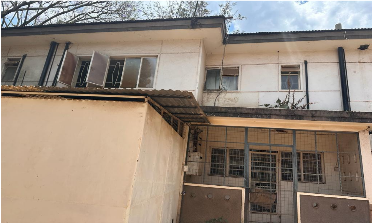
An existing Housing still in good condition
