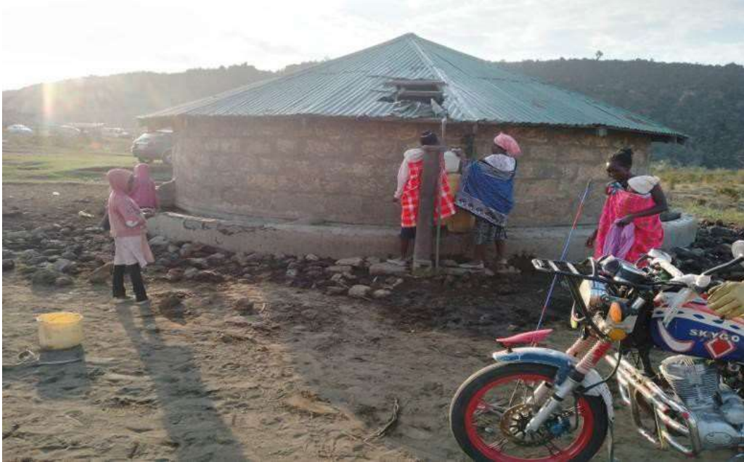
Figure 19: Olomayian water point
