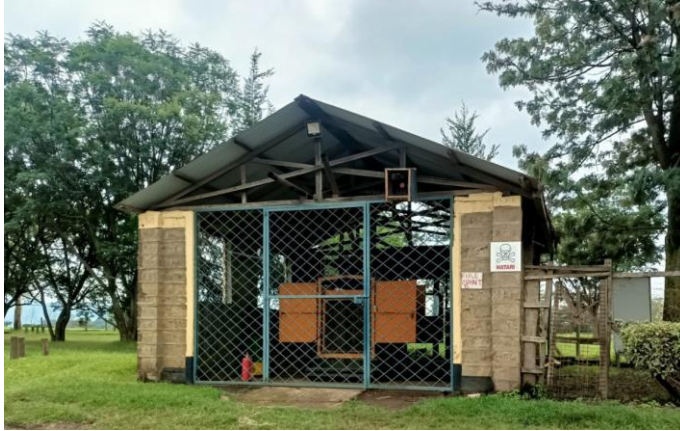
Plate 3: Existing generator room
