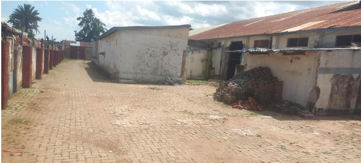
Figure 3.2: Paved compound without vegetation at the proposed site
