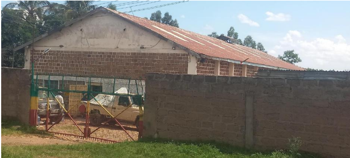
Figure 3.3: Another go down in the neighborhood to the proposed project site
