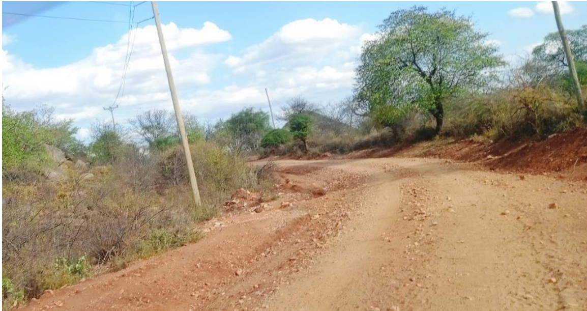
Plate 5: Sections of a feeder road that serves the proposed project area
