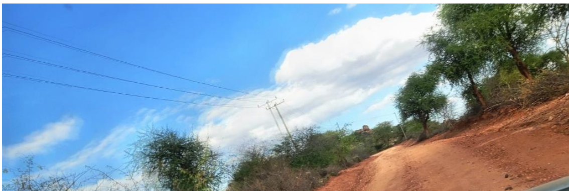
Plate 6: Power line supplying electricity to some sections of the project site
