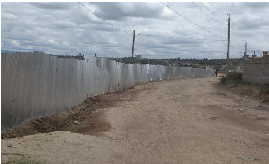
Plate 1: An adjacent access road that the proponent will modernize
