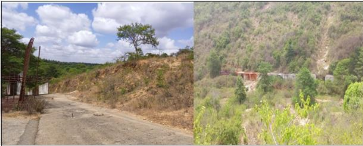
Figure 2: partially constructed concrete spillway and reinforced concrete diversion culvert
