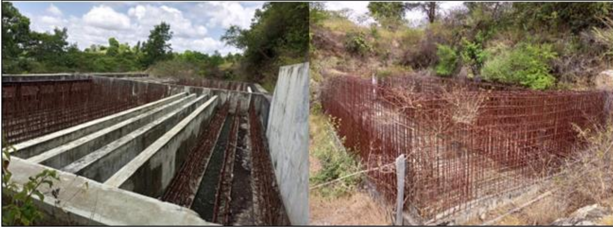
Figure 3:Partly constructed water treatment plant
