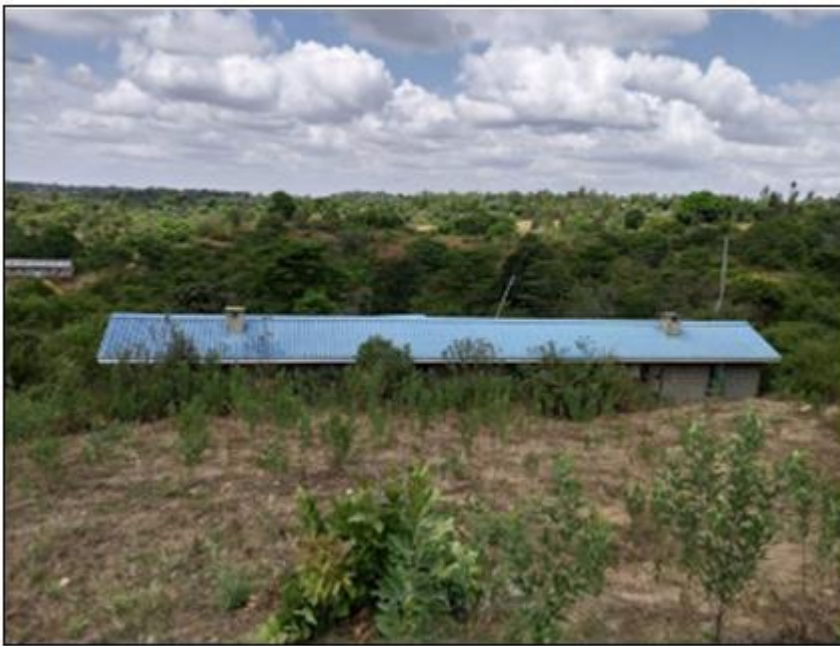
Figure 4:constructed Staff houses (only electrical works and finishes not completed)
