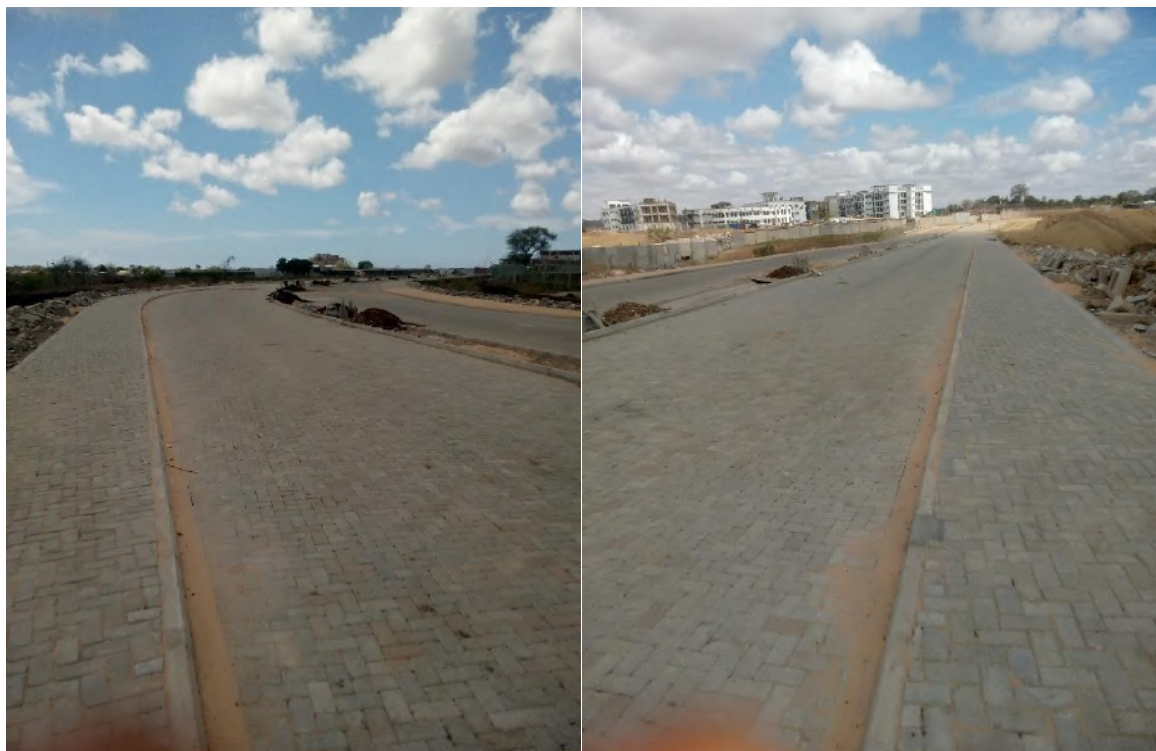
Fig 7.1: The project site access cabro road (Source, Site visit/photography)
