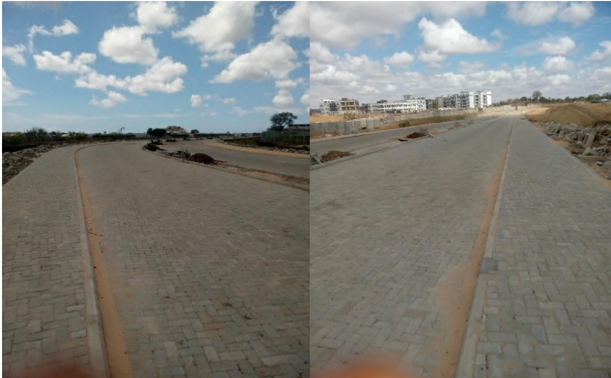
Figure 1.3: The project site access cabro road (Source; Site Survey/photography)
