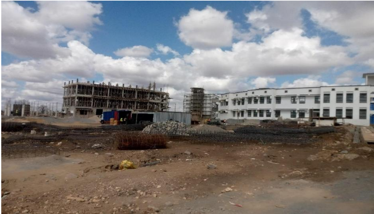
Fig 4.1: The ongoing project activity (Source, Site visit/photography)
