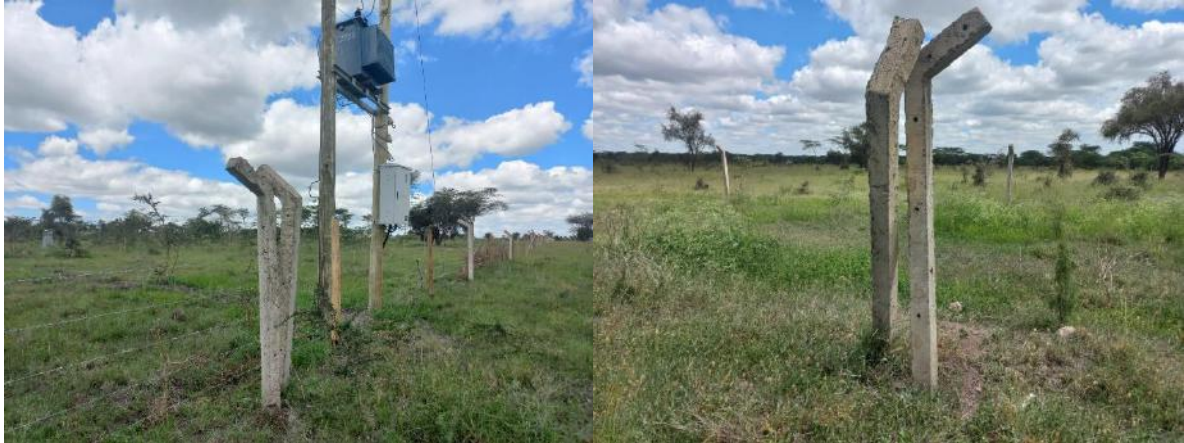
Poles used to demarcate the boundaries between the project site and neighboring parcels of land
