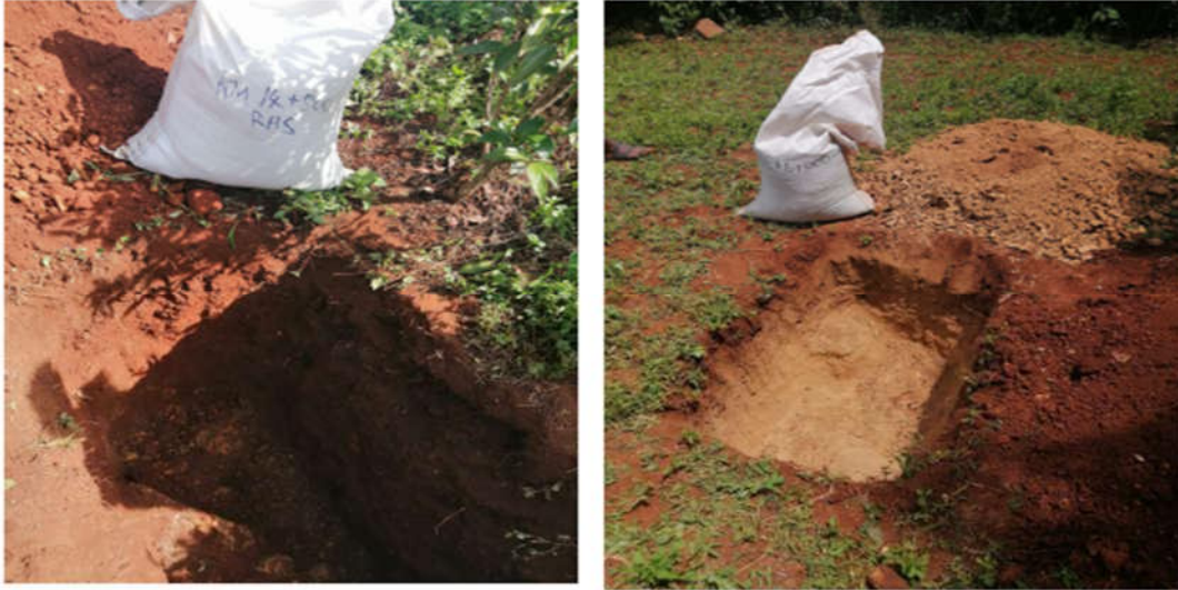
Plate 5: Sample alignment soil investigation trial pits
